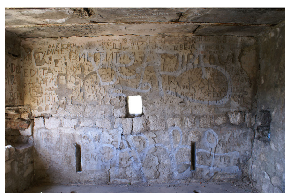
EXISTING LAYERS OF PLASTER
