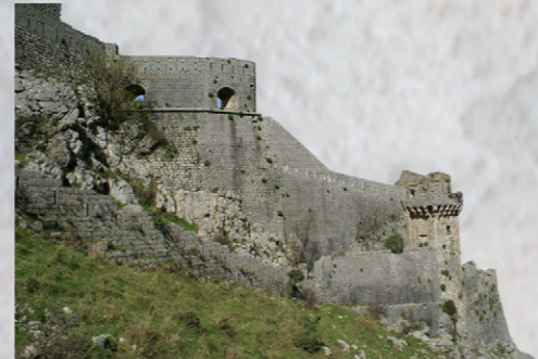
CONTARINI TOWER AND EASTERN CITY GATE
