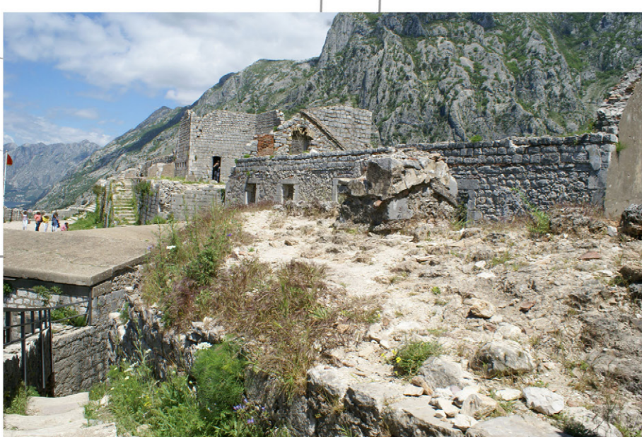
SAN GIOVANNI CHURCH ROOF
