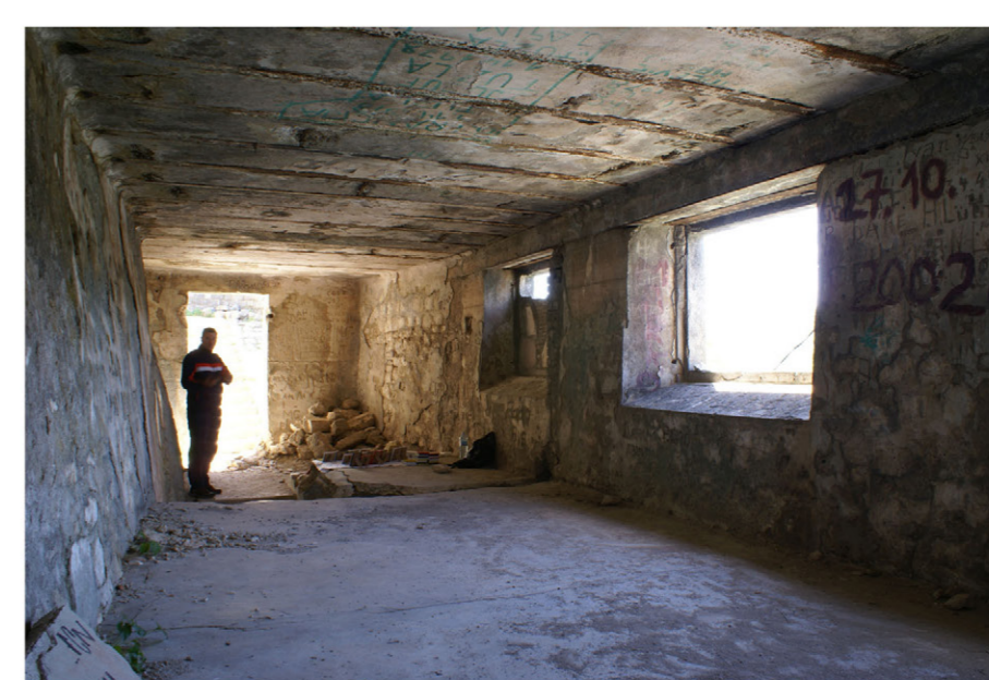
FIRST LEVEL INTERIOR VIEW
