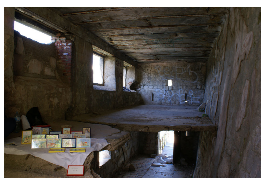
FIRST LEVEL INTERIOR VIEW
