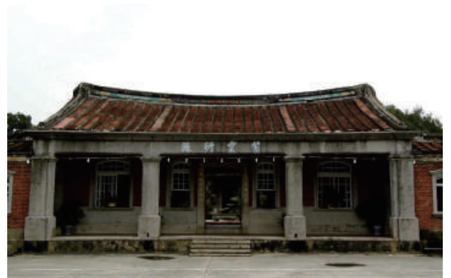
Historic building of Minnan migration Houbi Huang Family Mansion
