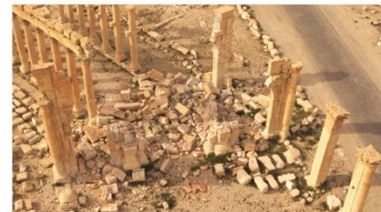
Aerial footage showing the damage of the Triumphal Arch - Source: DGM
