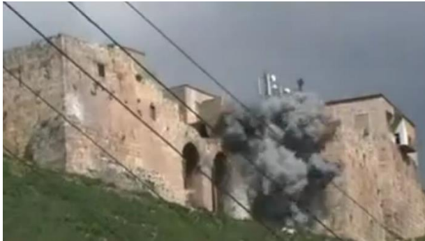
Shelling damage to citadel (15 March 2012) (Irina Bokova, 2012)
