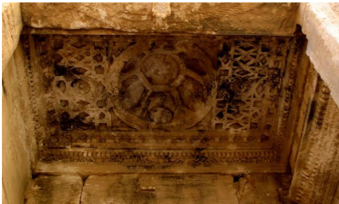
The Southern Roof, Photographer: Hisham Zaweet
