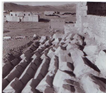
Temple of bel, Restoration work on the west wall - Source: SOAM
