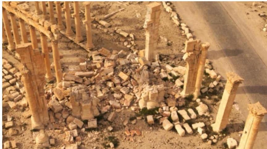
Ariel Footage showing the damage of the Triumph Arch (Museums, 2016)
