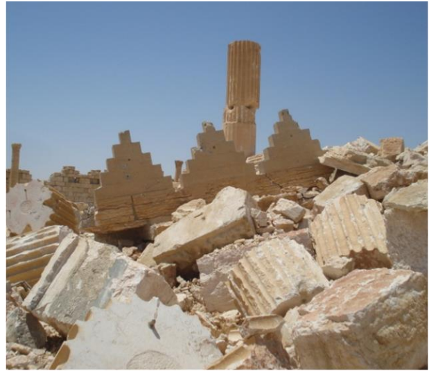
The Temple of Bel after ISIS destruction / The damage of the gate base, Source: Rania Al-Fahl
