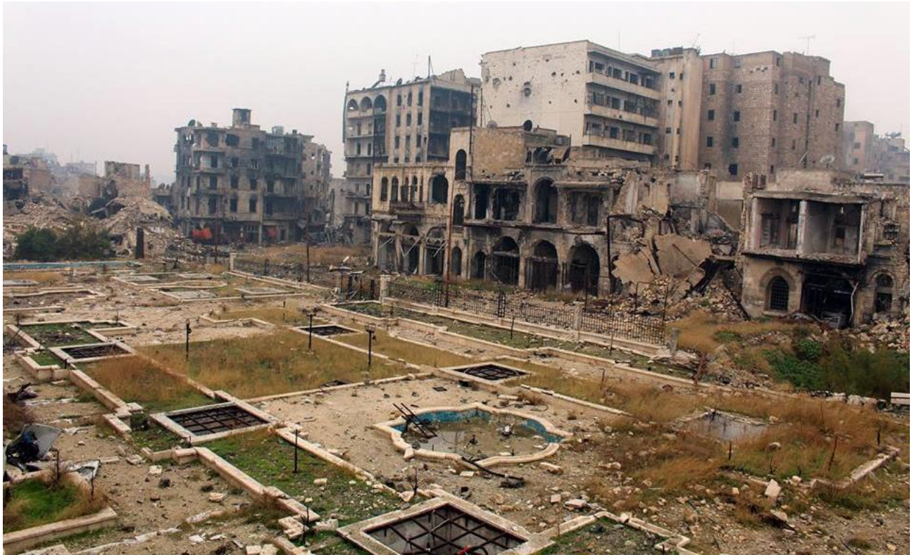
The damages in the piazza in front of northern entrance of the Umayyad Mosque Source: DGAM
