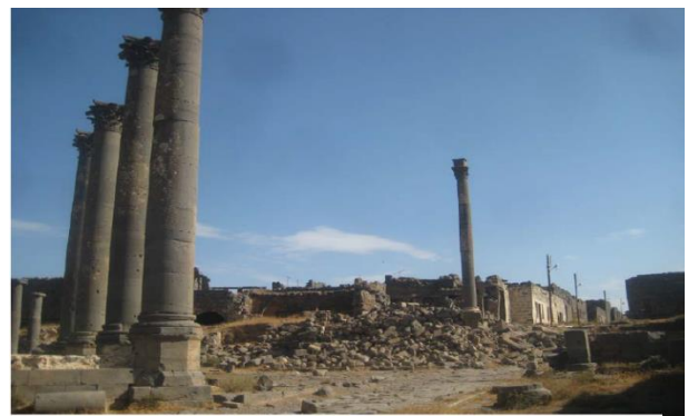
Severe damage to Kalybe, Cradle of The King's Daughter in Bosra, Source: DGAM 2014
