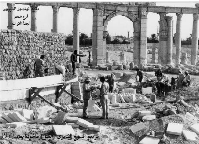
Restoration work on the theater / source: DGAM
