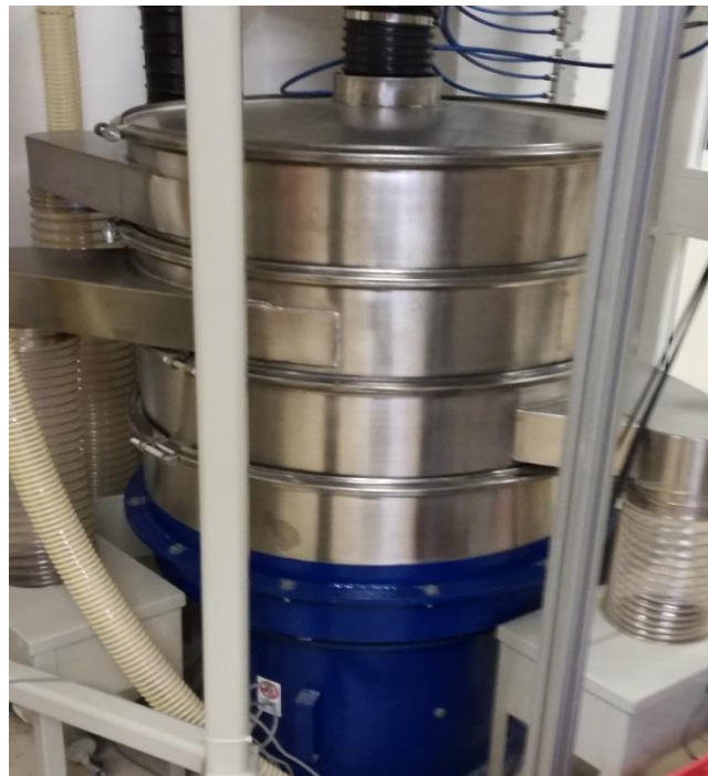
Figure 4.3: Vibrating separator
