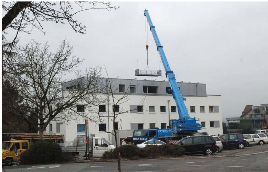
Figure 8 - Mounting of pre-fabricated balconies
