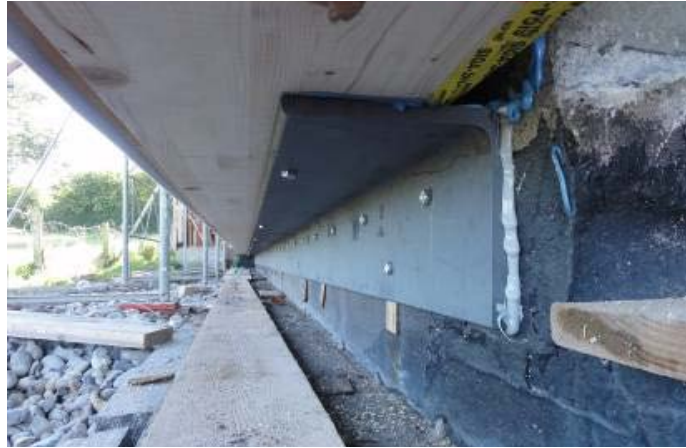
Figure 6 - Horizontal mounting angle and a modules just before its final position
