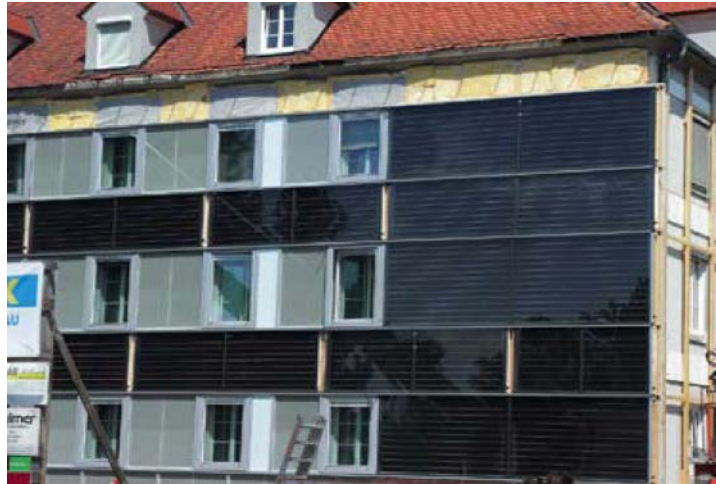
Figure 9 - assembly of the modules on the south oriented facade
