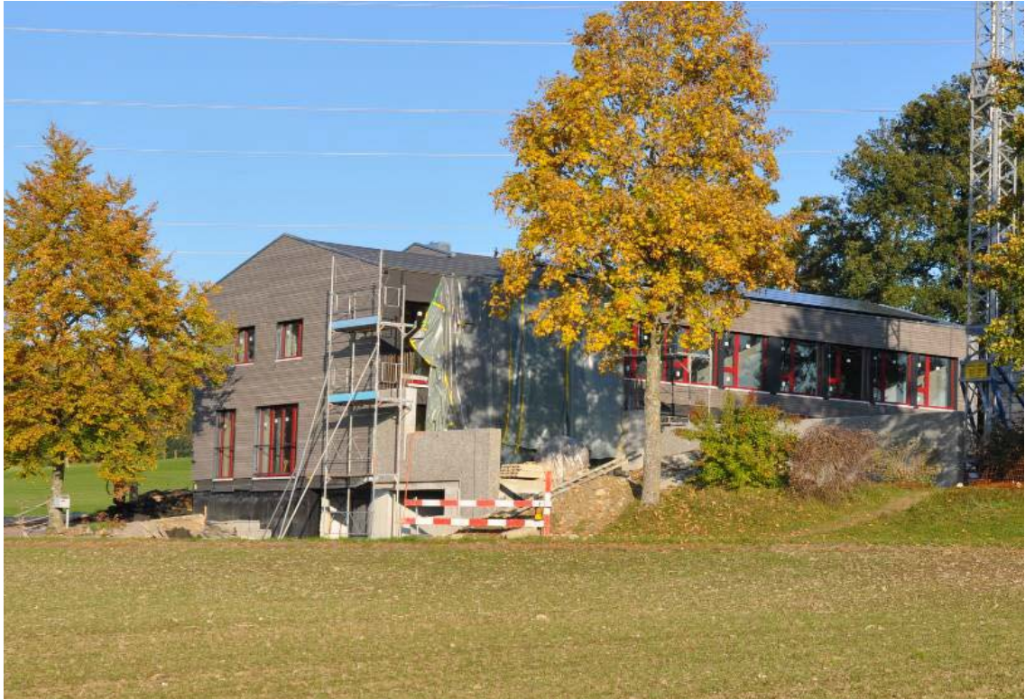
Figure 9 - View of renovated building just before completion
