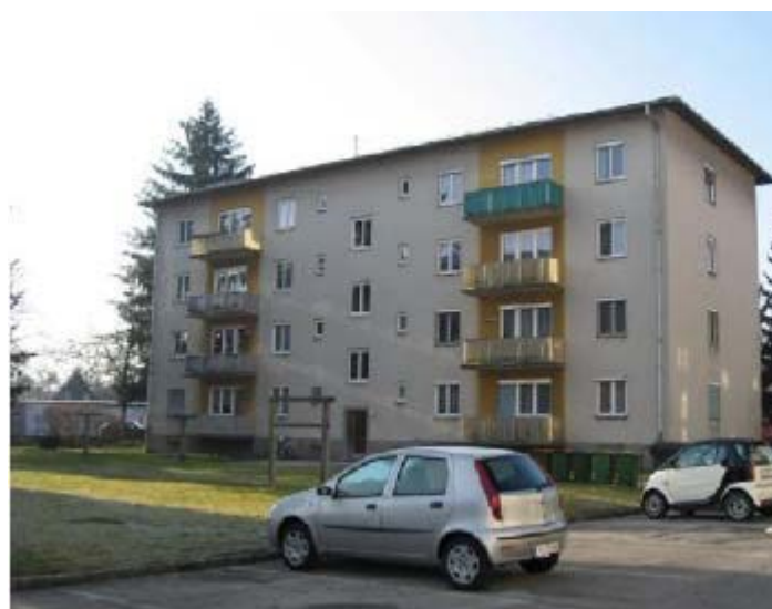
Figure 1 - View of apartment building before renovation
