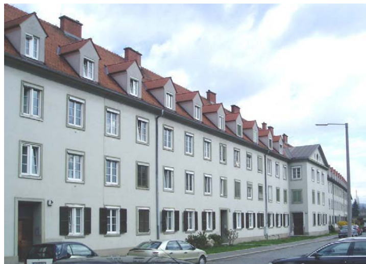
Figure 1 - View of apartment building before renovation
