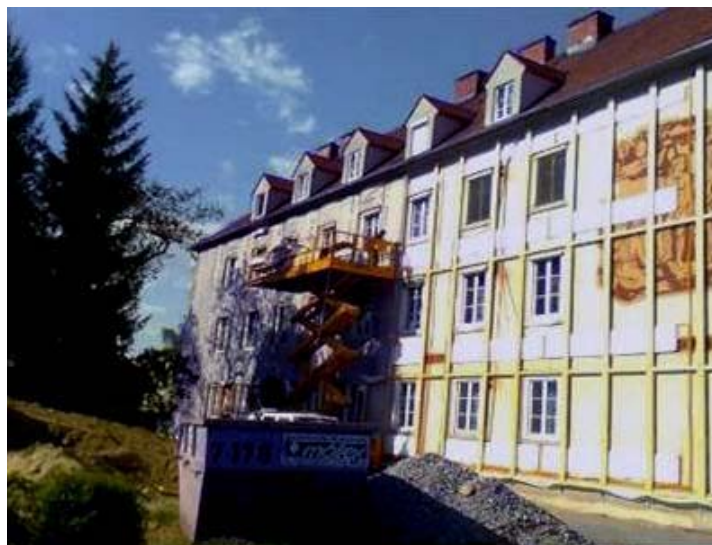
Figure 6 - Heat distribution and XPS-boards are installed on the existing facade
