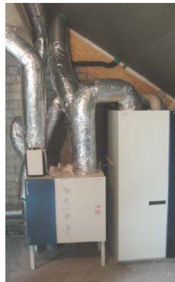
Figure 6 - combined heating, ventilation and DHW system
