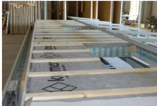
Figure 8 - Preparation of the timber frame
