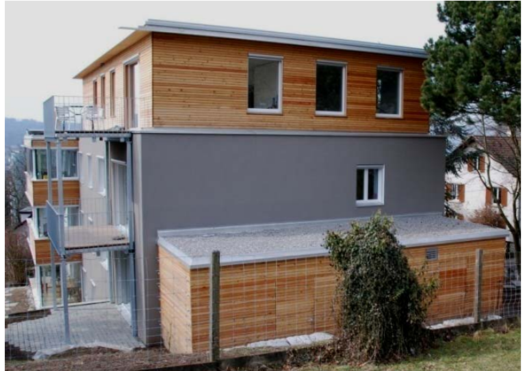
Figure 5 - Renovated building from the north-eastern side. The building annex is used as technical space for the new heating system (ground coupled heat pump)
