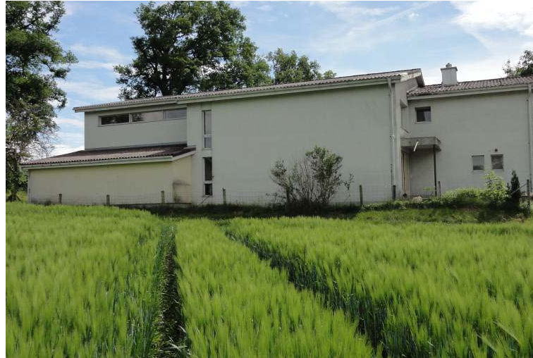
Figure 1 - View of old building and project
