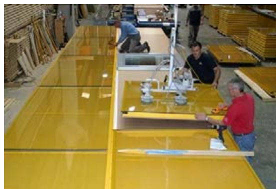
Figure 9 - Solar comb installation (source Gap-Solutions)
