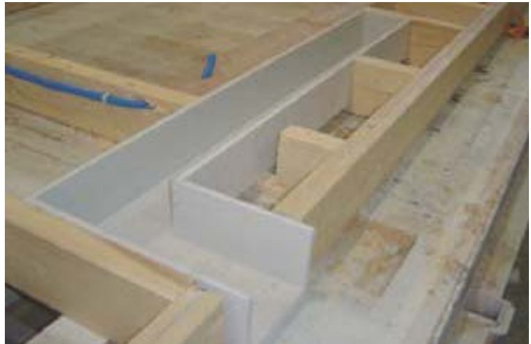
Figure 6 - Factory assembling of façade module with fire proof ventilation cavity
