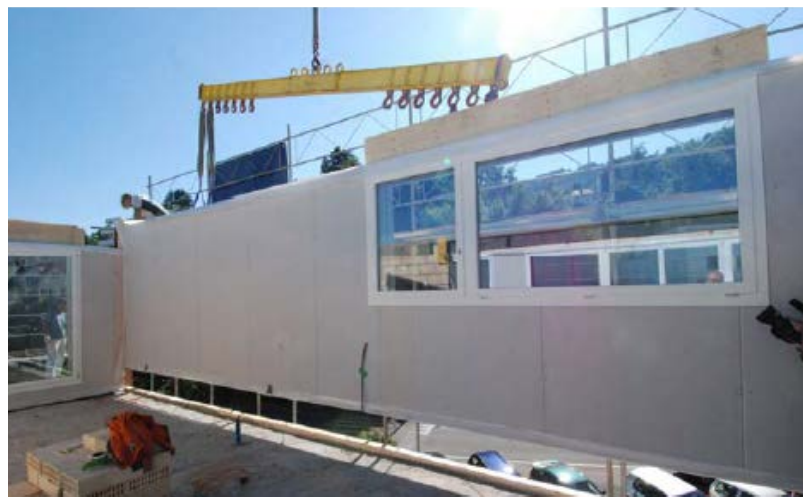
Figure 5 - Mounting of the prefab structure
