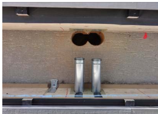
Figure 7 - ventilation ducts integrated in the prefab module
