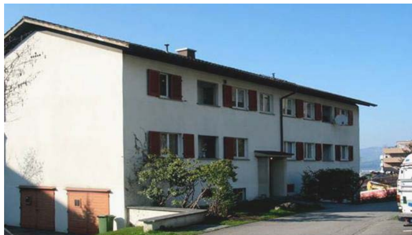
Figure 1 - North-east view of apartment building before renovation
