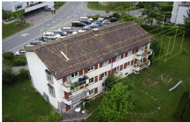
Figure 2 - View of old building and project
