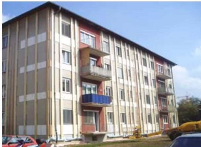
Figure 6 - Heat distribution and XPS-boards are installed on the existing façade
