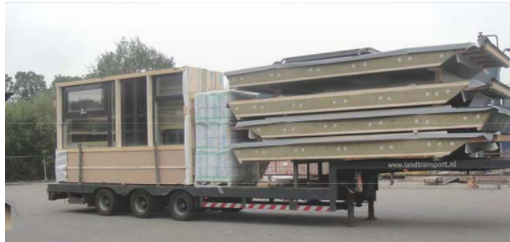
Figure 7 - Transportation phases of the prefab element
