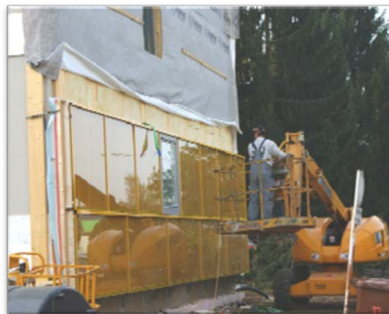
Figure 10 - Assembly of the lowest module
