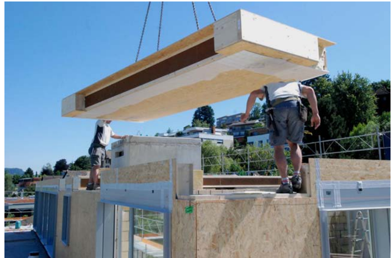
Figure 6 - Mounting of prefabricated roof elements for new attic apartment
