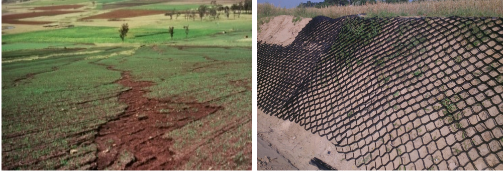
Figure 2.4: Sheet erosion with rills forming in the background(left) and a stabilizing geosynthetic (right)
