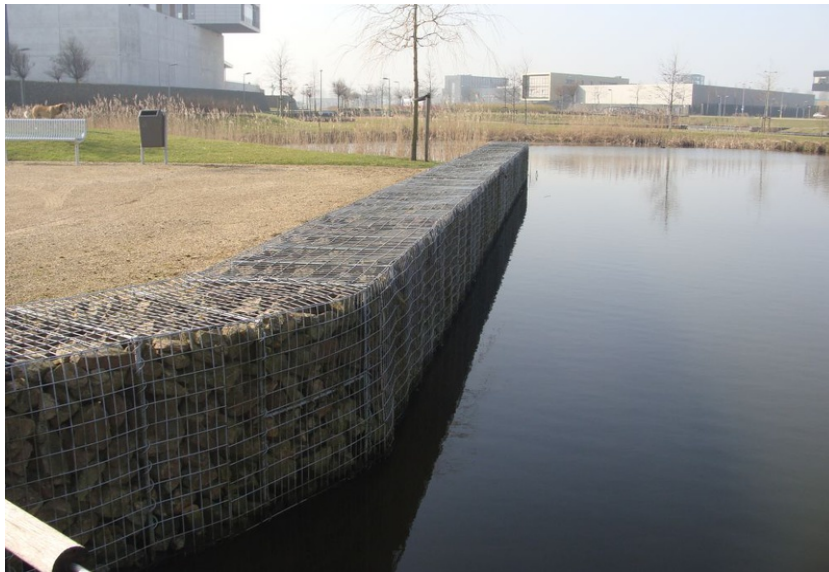
Figure 2.12: Riverbank protected with gabions
