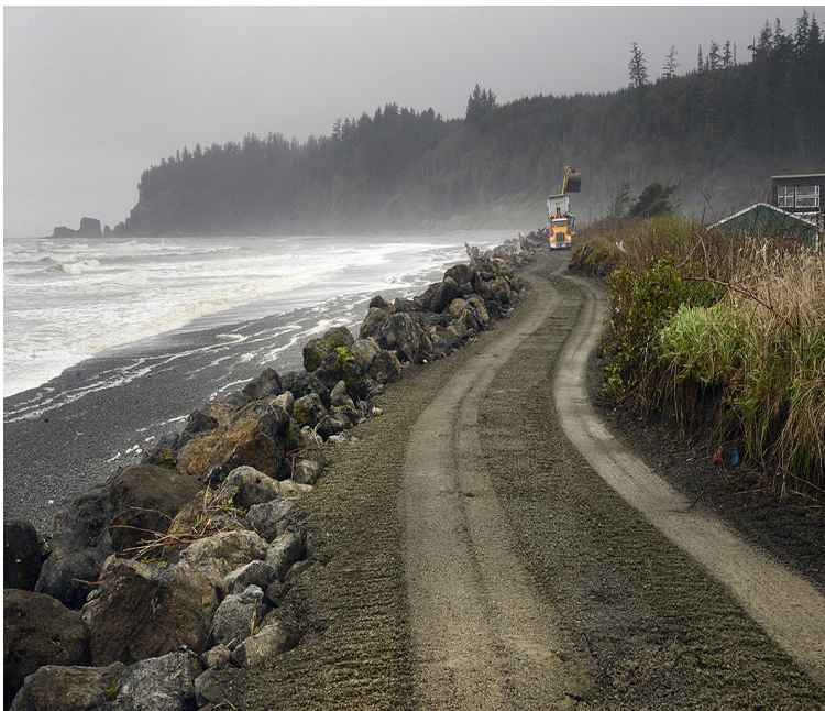
Figure 2.8: A stony seawall
