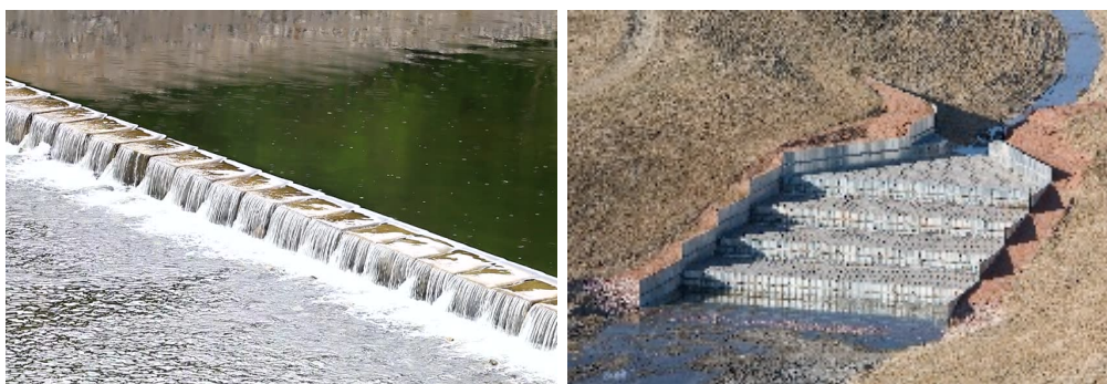
Figure 2.13: A checkdam (left) and a drop (right)
