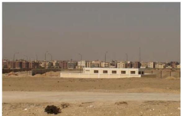
(06) Electrical plant facing the site
