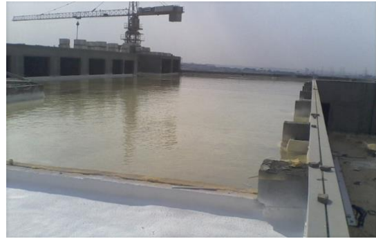
(6) FLOOD TESTING THE ROOF
