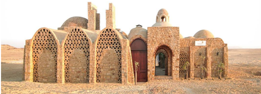
Fig. 3.13 Traditional and vernacular buildings
