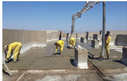
(2) PANELING AND SCREED LYING
