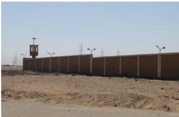
(05) Electrical plant area
