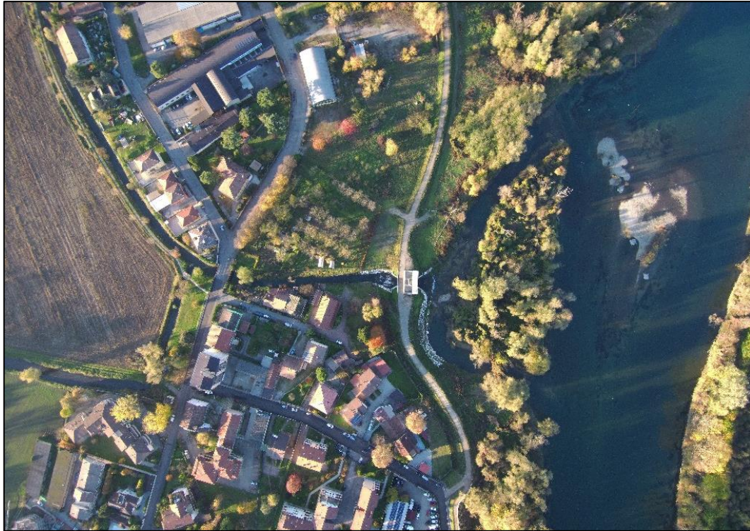
Figure 19 Photo of drone survey
