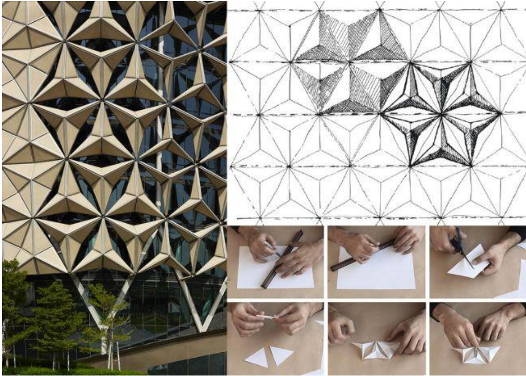
Figure 18 - Example of kinetic facade, Al Bahar Towers, Abu Dhabi. Image credit to http://www.infobuildenergia.it/progetti/al-bahar-towers-torri-abu-dhabi-facciata-solare-intelligente-477.html
