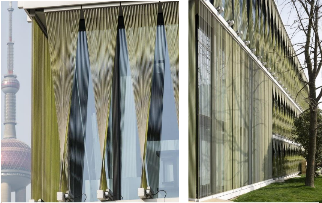
Figure 50 - External views of the dynamic shading (photo credits to Bartosz Kolonko)
