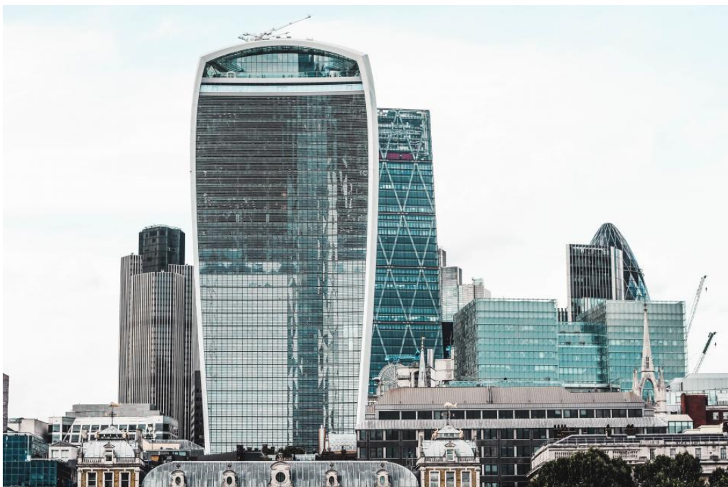
Figure 16 - Typical architectural features involved in the design of today's commercial buildings: the provision of high WWR is very common and widespread all over the world. Free stock image, last accessed March 23, 2018; https://stocksnap.io/photo/YWJJ8BCZE4
