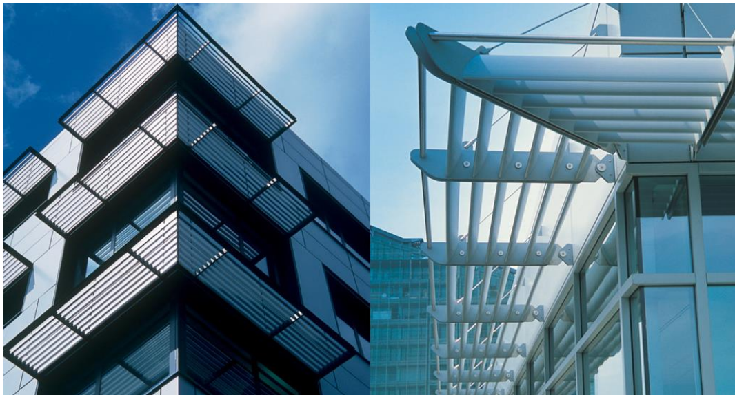
Figure 13 - Example of a typical fixed shading consisting in a horizontal louver. Image from Archdaily.com, last accessed March 22, 2018; https://www.archdaily.com/catalog/us/products/11876/solar-shading-reynaers-aluminium/111493
