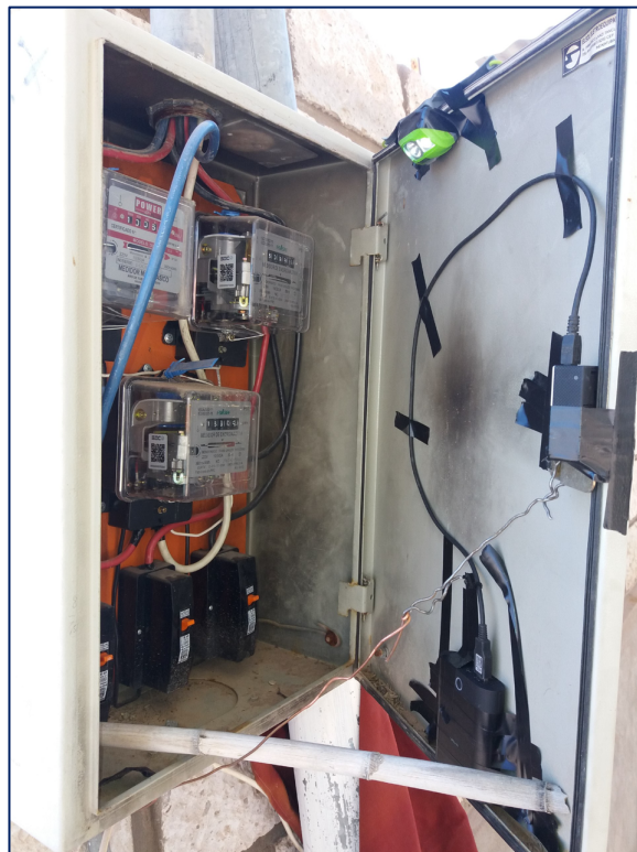
Figure 5: Camera installed to monitor energy consumption of the local Public School. Source: Authors.
