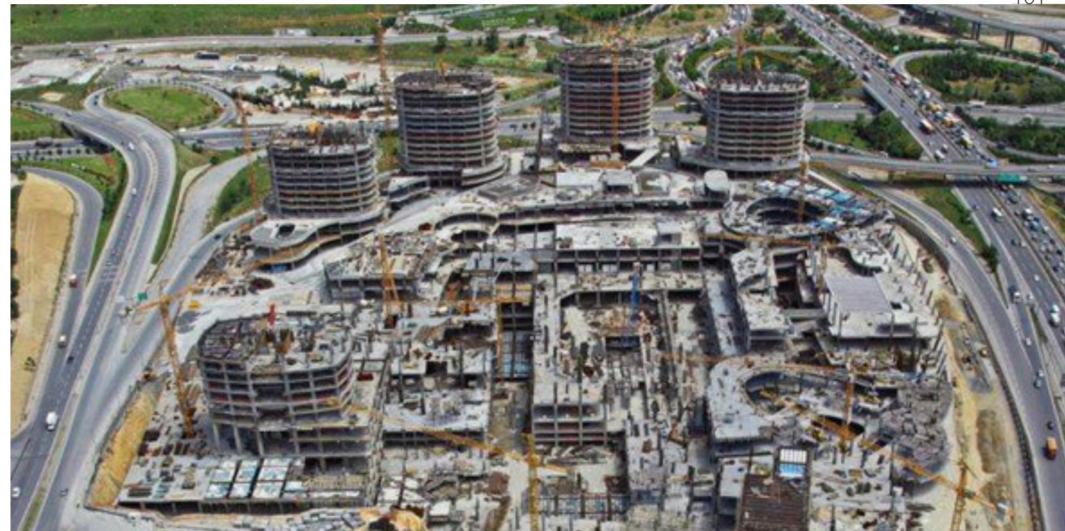
Figure 41. Mall of Istanbul Construction Aerial View. June 2012.
