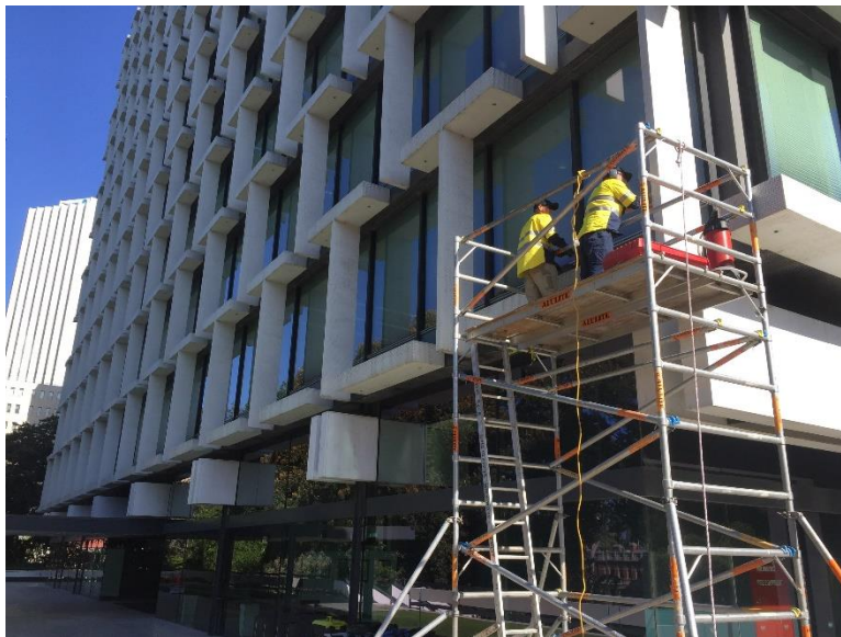
Figure 34 - Facade Inspection - Source: MEnD.com
