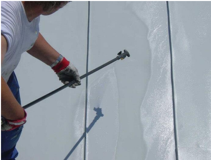
Figure 36 - Facade Protection and Treatment - Source: hseintegro.com
