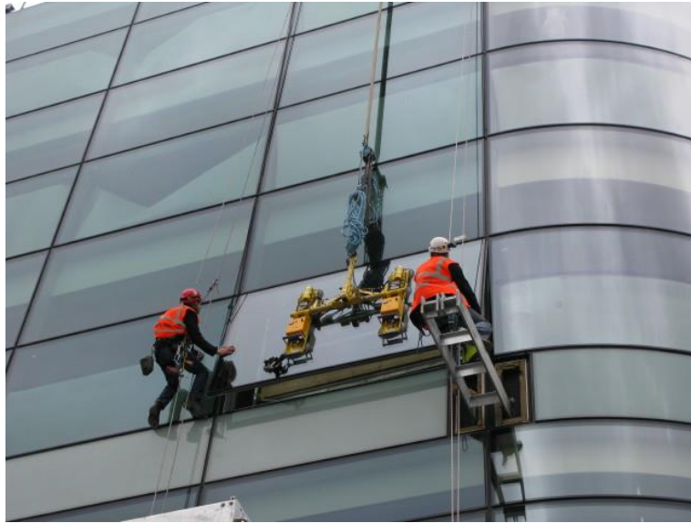
Figure 37 - Façade Replacement - Source: Constructionweekonline.com
