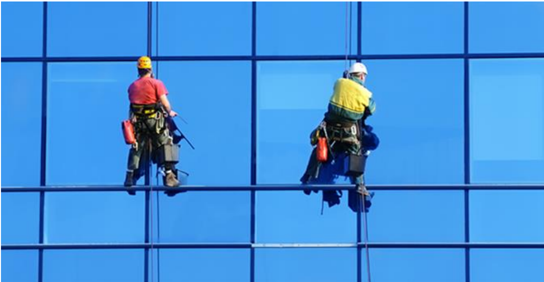
Figure 35 - Facade Cleaning - Source: Hseintegro.com
