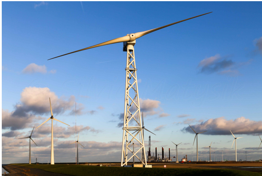
Figure 1.4: Modern two blade 2-B 2B6 wind turbine.
