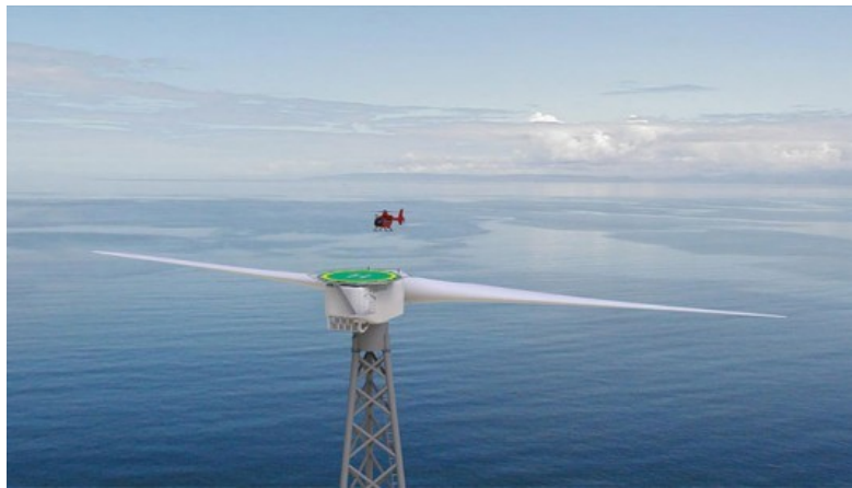
Figure 1.2: 6MW two-blade wind turbine.
