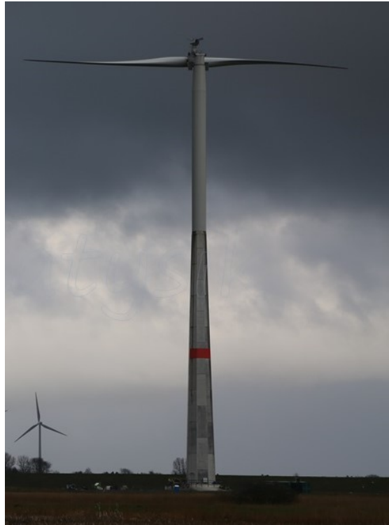
Figure 1.5: SkyWind 3.4 MW wind turbine, rotor diameter 107 m.
