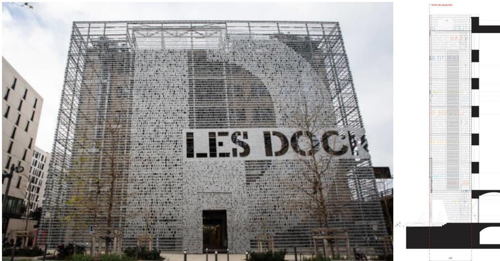
Figure 2.29 Northern façade covered and opened - Source: Constructa Urban Systems, 2013, Les Docks Roadbook Version 2.0
