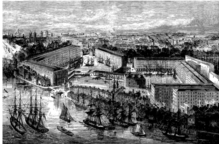
Figure 2.5 St Katherine's Docks, London, built in the 1830s – Source: www.british-history.ac.uk
