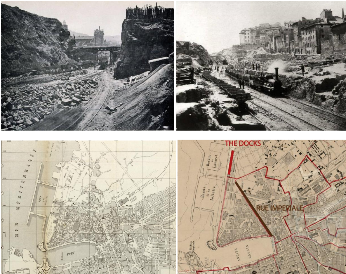
Figure 2.4 Up Left: Sadie Carnot hillock pierced during Rue Impériale works. Up Right: Rue Impériale dug. Down Left: Marseille in 1852, La Joliette basin planned, but no Rue Impériale yet. Down Right: Marseille in 1862, other basins added, Rue Impériale dug – Source: photos and basemaps from Marseille Archives.
