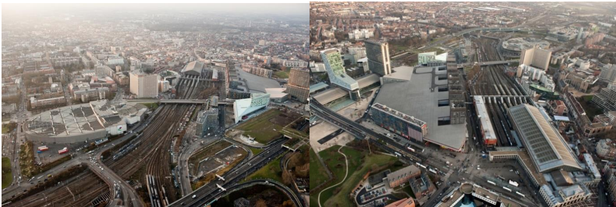
Figure 4.6 Two points of view on Euralille around the high-speed railway station, Lille – Source: OMA.
