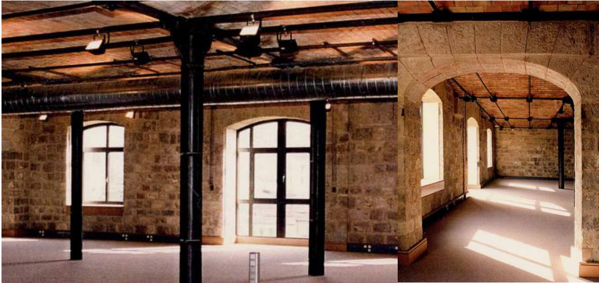
Figure 2.19 A finished open space. Cast iron pillar painted black and completed by dark iron light holders, historic materials valorised – Source: Castaldi Archtecte.
