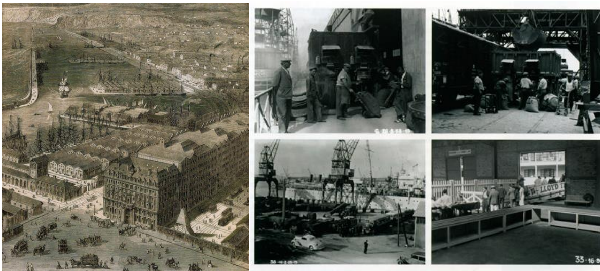
Figure 2.10 The Docks in the 19th century: cranes and smaller storage buildings on La Joliette quay, activities inside the building - Source: www.les-docks.fr
