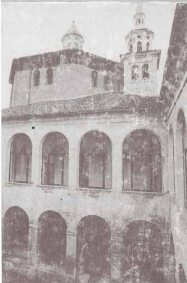
Fig 14: The inner façade of the courtyard of Incoronata church. The inner loggia can be considered an example for the reconstruction of the armory in Piazza D'Armi
