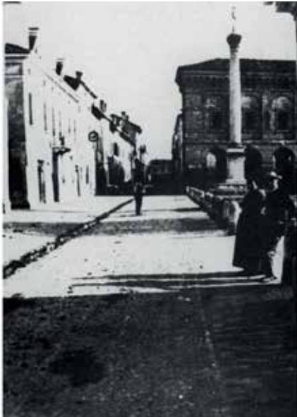
Fig 2: Sabbioneta, Via Giulia (today Via Vespasiano), before the paving in porphyry, end of XIX century, Archivio storico comunale
