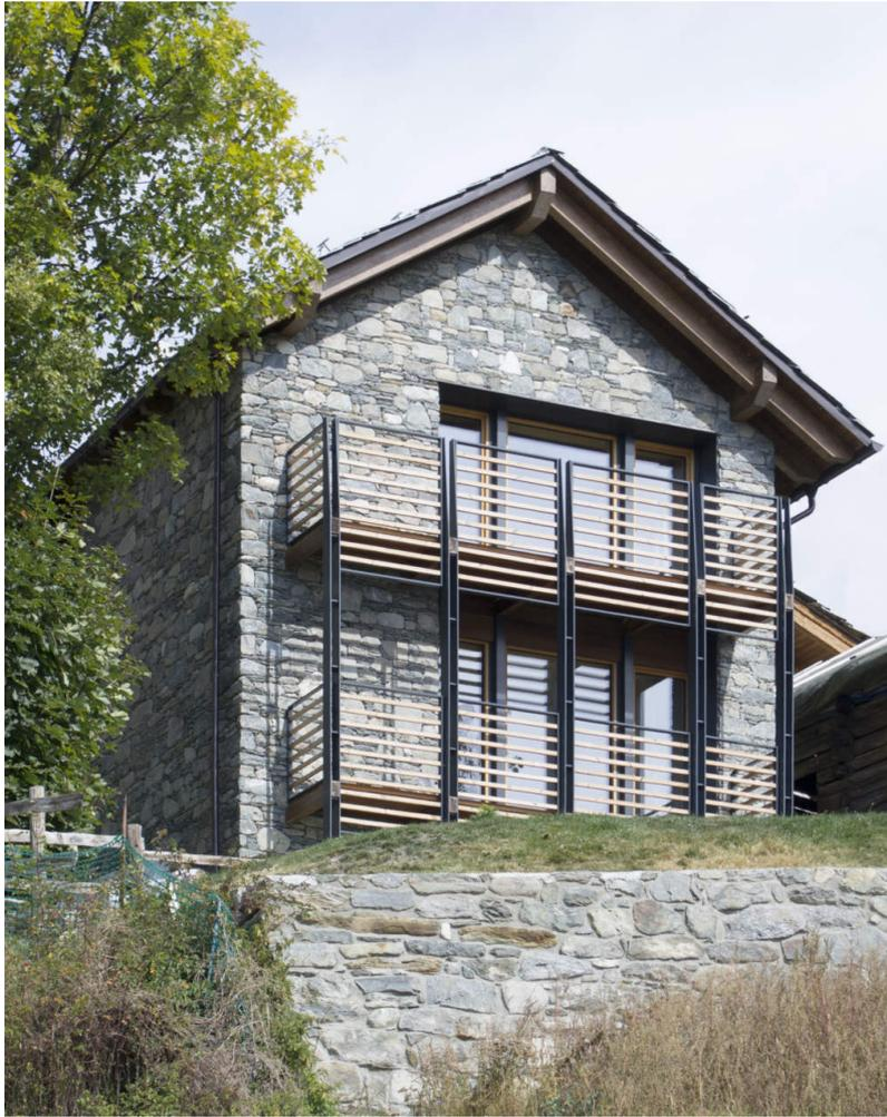
The whole house is made mainly with pre-fabricated materials, that are assembled in situ with completely dry method; this reduces the construction time and the polluting emission. This is a load-bearing wooden wall infilled with straw, that both reduces the transmittance and naturally regulates humidity.
