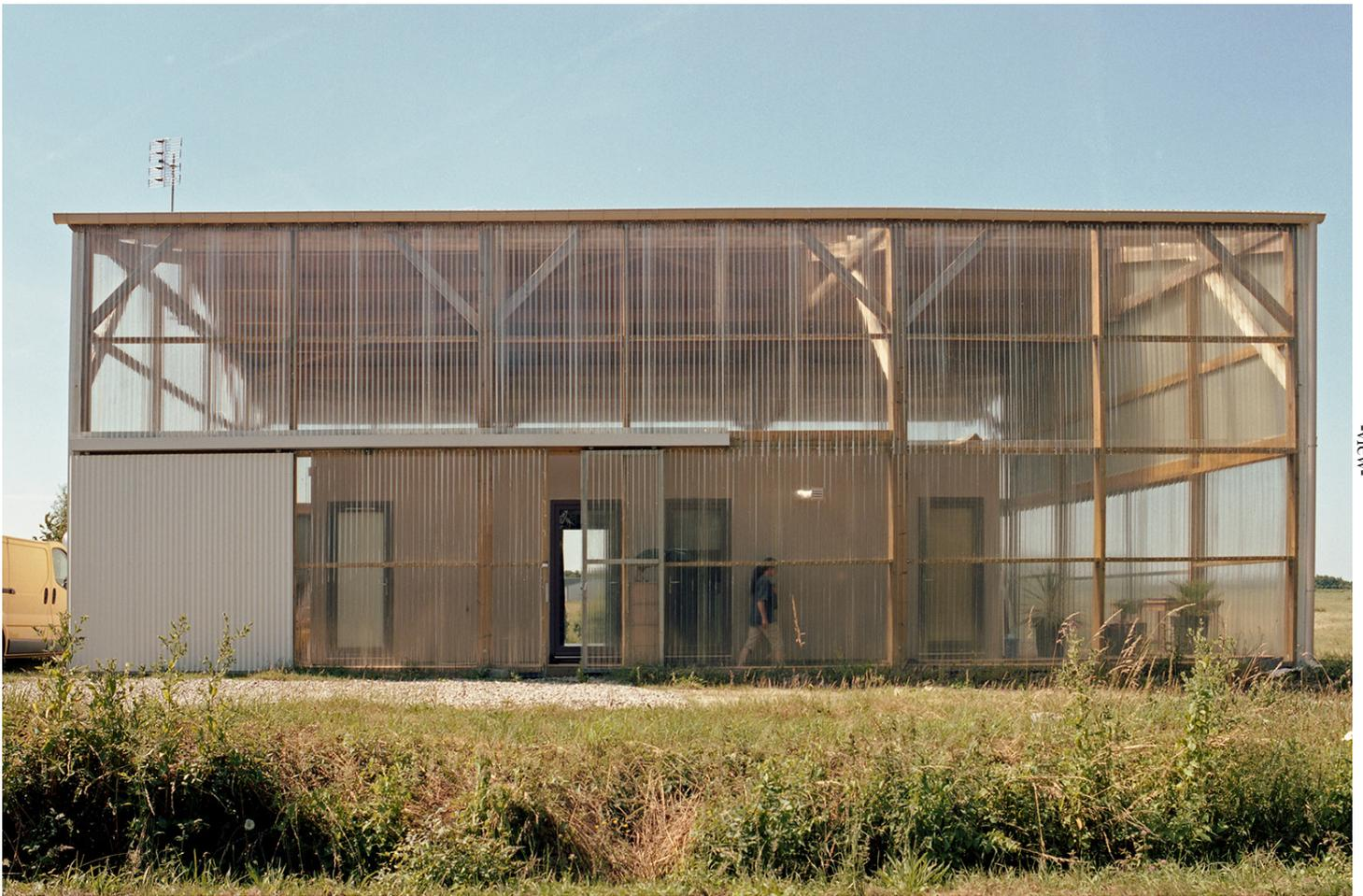
Constructively the complex is made by essentially two detached elements, the house and the framework. The last one is designed to reduce the energy requirement of the building, shading the sun in the summer and allowing hot air to easily flow over the house, and creating greenhouse effect in the winter thanks to the polycarbonate panels.
