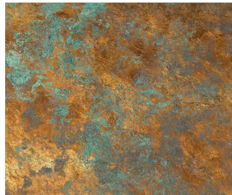
Copper partially oxidated.
