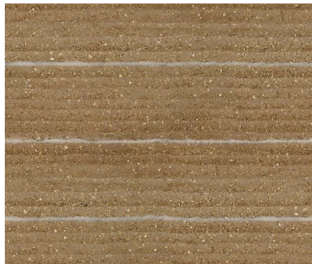
Pisè technique, earth walls.
