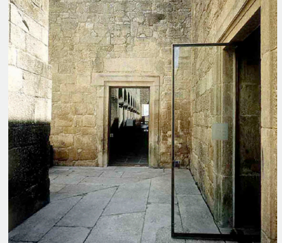
Fig. 86_Pousada de Santa Maria do Bouro, Souto de Moura: Veduta della corte Fonte: https://images.adsttc.com/media/images/5583/988e/e58e/ce09/c200/00bf/large-jpg/5.jpg?1434687624
