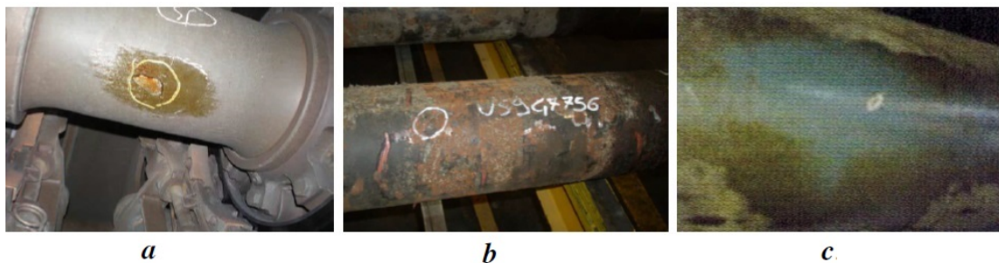
Figure 2.9: Examples of in-service railway axle damage.
