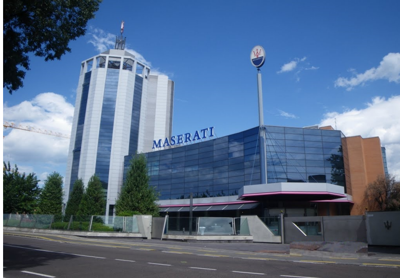
Figure 1.3: Maserati's headquarters in Modena, viale Ciro Menotti 322
