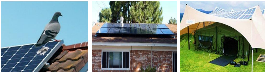
Figure 2-4 Partial shadow conditions on photovoltaic panels
