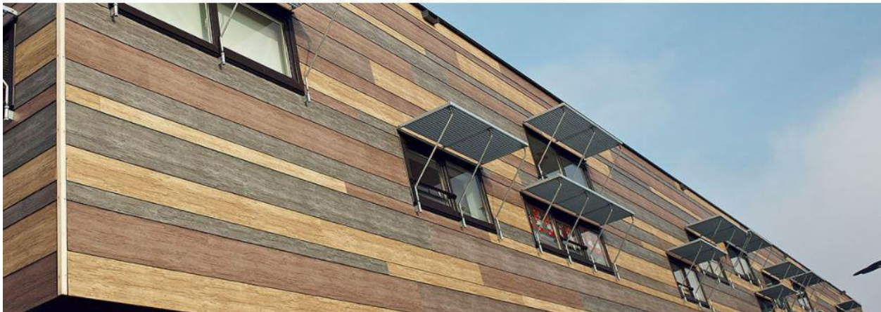
Fig. 5.6.1. Rockpanel Woods Façade Example
