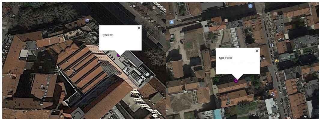
Figure 5.19: Type 7 substation in google map
