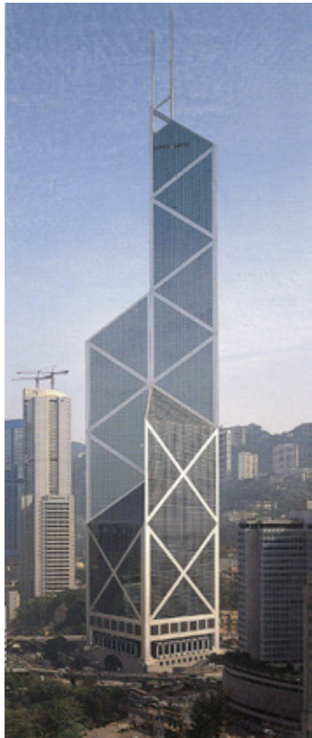
Bank of China Tower, LM.Pei & Partners Hong Kong, 1990, 367,4 m
