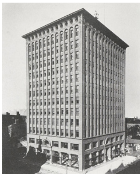
Guaranty Building, Dankmar Adler & Louis Sullivan, Buffalo, 1896
