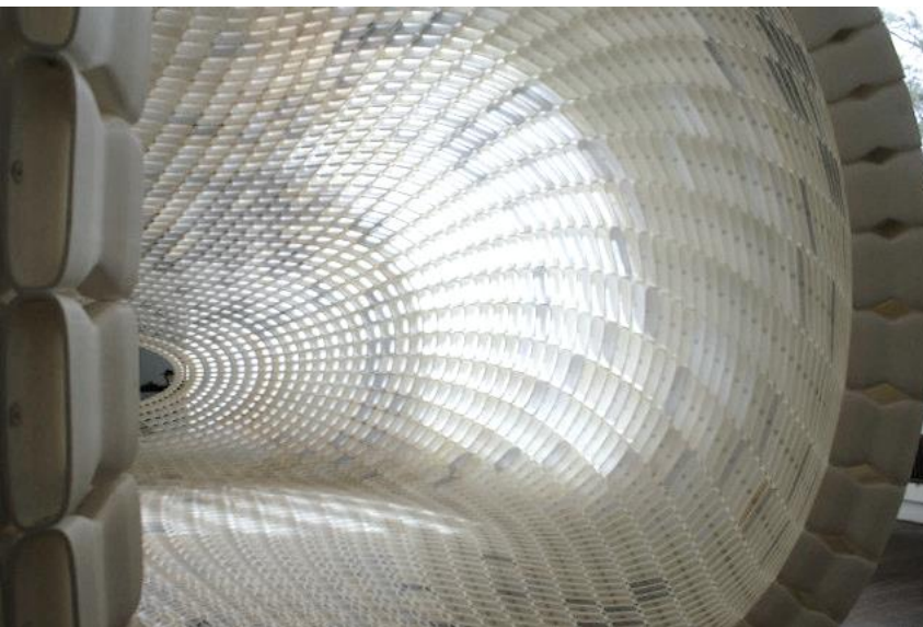
Egg-Shaped Pavilion, world's largest collectively 3D printed project by Dutch designer Michiel van der Kley,, Project EGG uses biodegradable polylactide (PLA) plastic. (2015)
