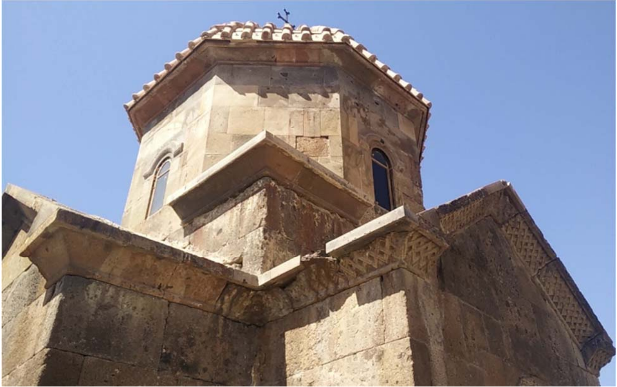
Surb Sion Church in 2017. A new stone dome is reconstructed. Photo by Samvel Martirosyan, September 2017.
