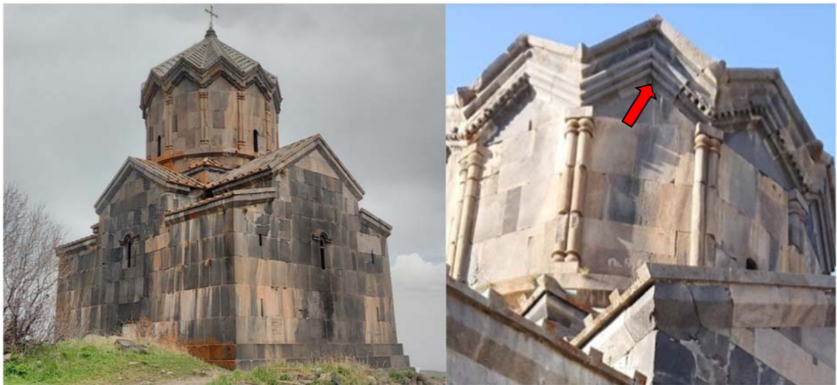
Left: The current situation of Amberd Church. Right: Highlighting the difference between the original and new stones by using plain, not decorated stone blocks. Photo taken by Vahe Simon in May 2017.
