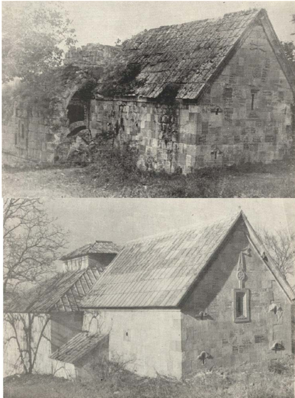
Mshkavank, before and after the restoration project of 1955-57. The broken and missing stone blocks were replaced and the cornices and roofs were restored.
