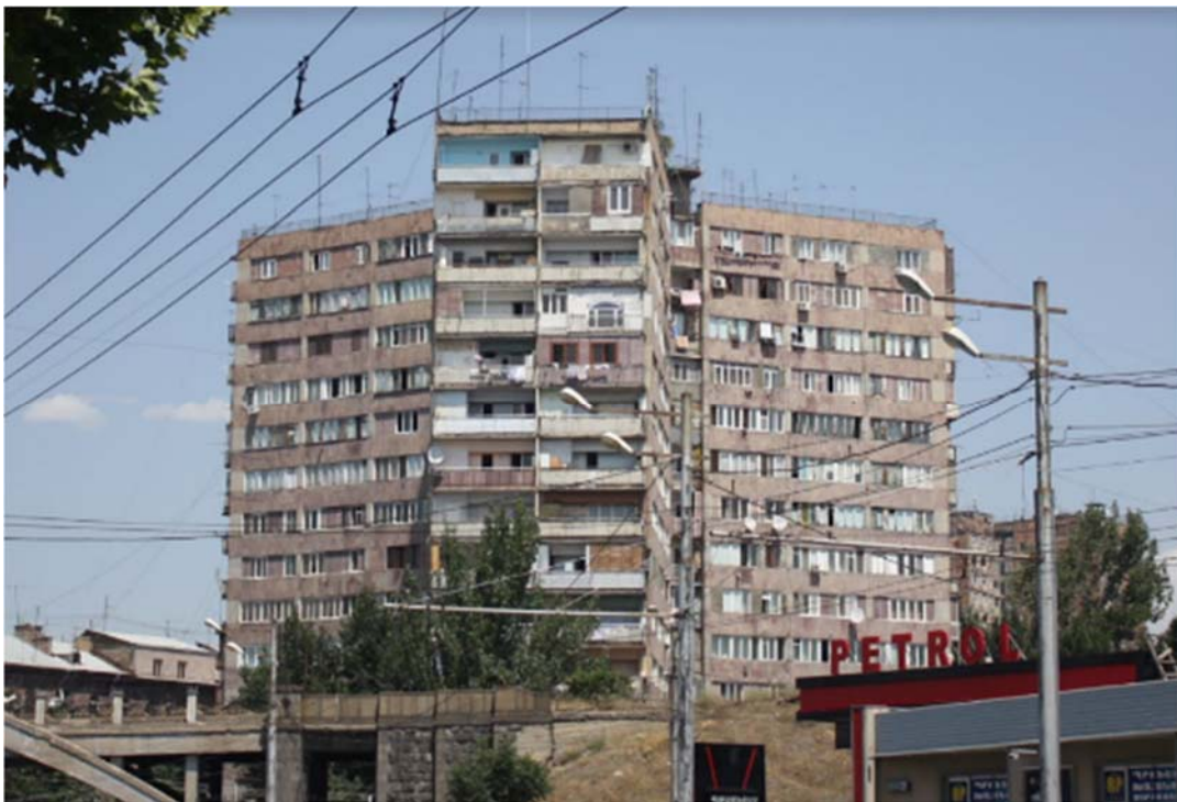
A high-rise residential building in Yerevan. Photo taken by author in August 2014.
