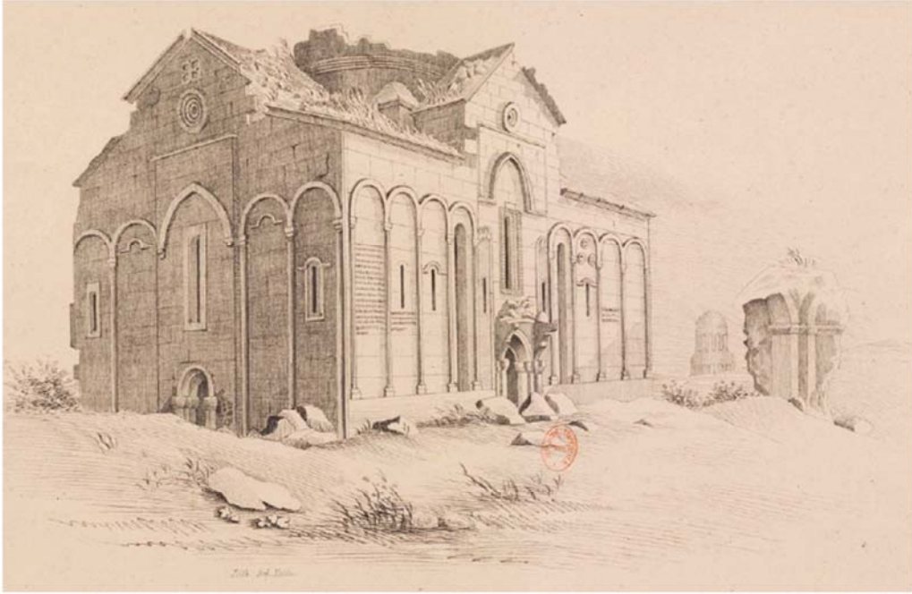
Figure 12: Ani cathedral, by Brosset, 1860. The state of preservation is clearly visible. Although not a scientific survey, but there is no attempt to complete any damage. This category of depictions are valuable source to analyze the state of preservation in different time periods. From Brosset, M. Les ruines d'Ani: capitale de l'Arménie sous les rois Bagratides, aux Xe et XIe S, histoire et description. Eggers et cie, Saint Petersburg, 1860. Atlas General, 45 planches, plate VIII.
