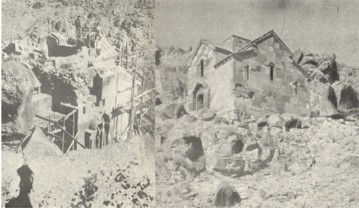
Saint Stepanos Church of Kosh before and after the restoration project of 1974-76. The pediments and upper section of the walls were heavily damaged and the dome system was totally lost. The pediments and missing stones were restored, the roofs were reconstructed and the first row of drum blocks were laid. The dome was not reconstructed because of unknown original form.
