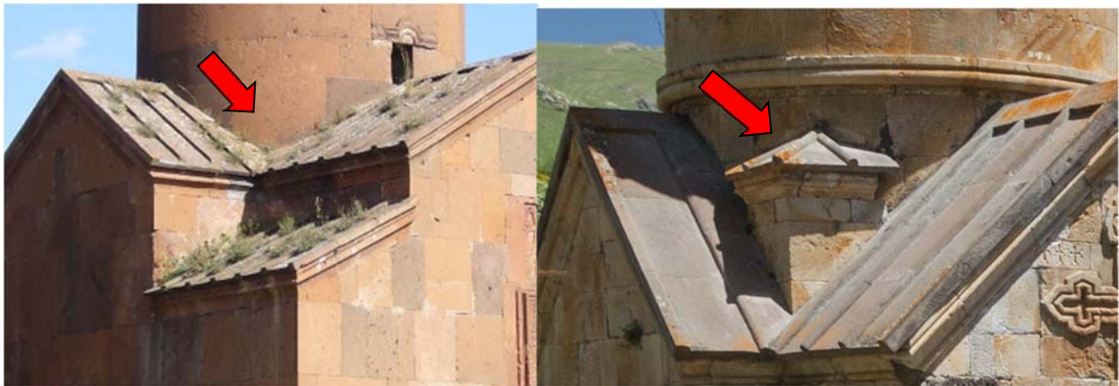
Left: A detail view of the southern church in Marmashen highlighting the missing common traditional Armenian architecture element. Right: An example of the above mentioned element.
