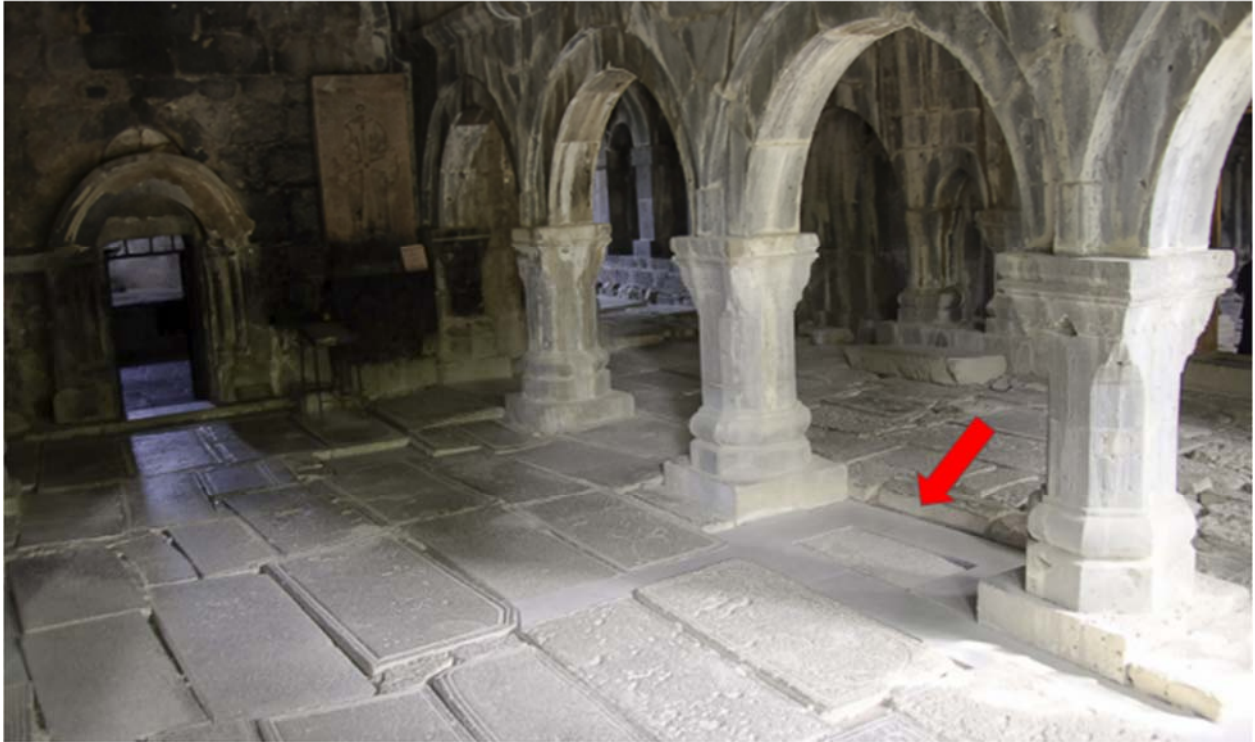
Isolating medieval tombstone, not perfectly level, will cause its rapid degradation by high number of tourists walking on them. Photo taken on 30 September 2016 by Diego Delso.
