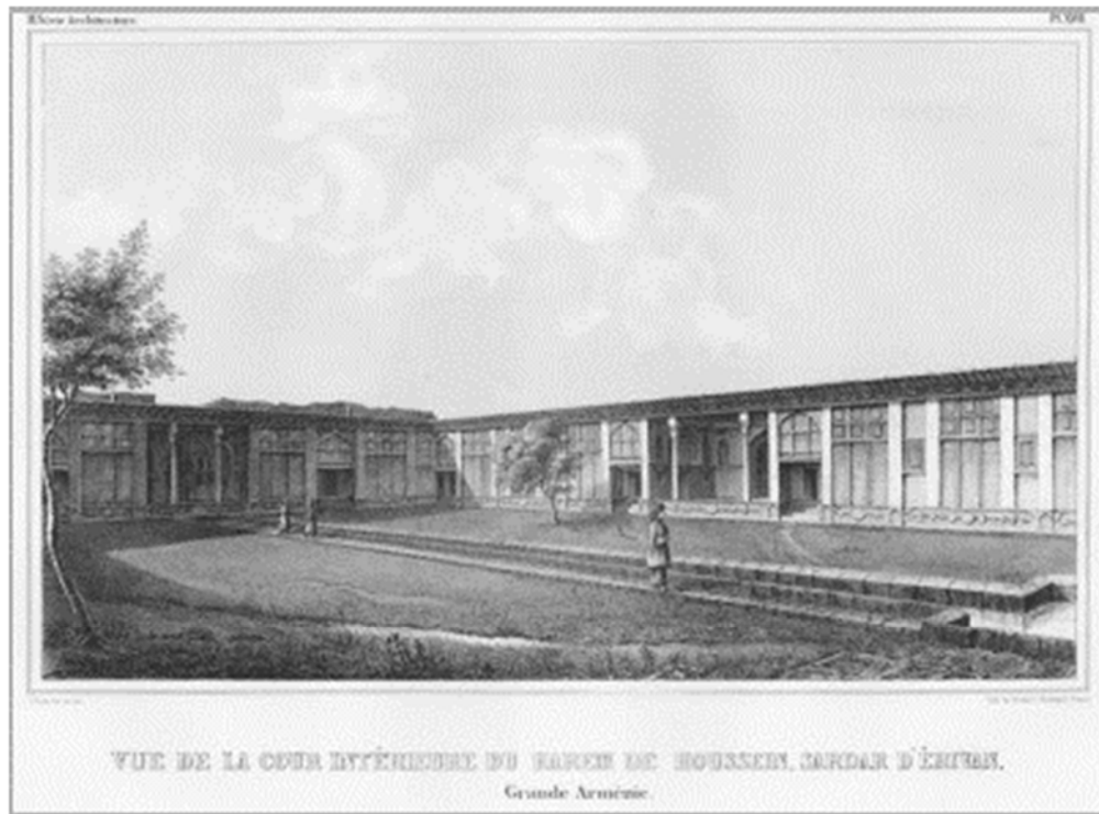
Figure 20: The inner courtyard of the harem of the Yerevan Sardar Palace, converted into a hospital. Illustration from Dubois, Atlas III, plate XXVII.
