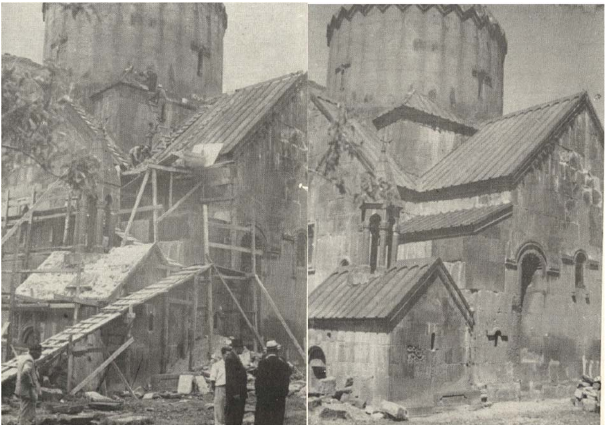
Bjni Holy Mother of God Church before and after the restoration project of 1957-59.
