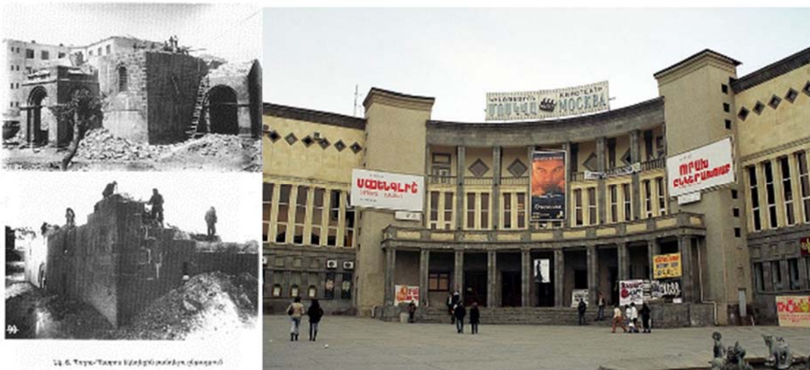
Left: Saint Paul and Peter Church during its demolition in 1930. Right: Cinema Moscow Building a after its restoration in 2000.
