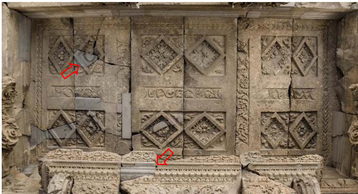
Figure 31: A photograph of the ceiling of the Garni temple highlighting the original and new stones. Photo by Author.
