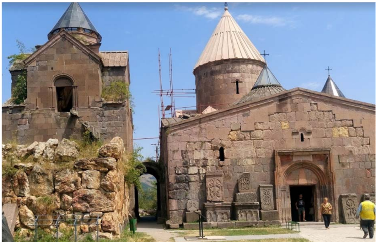
Goshavank in 2017. The main dome is recently covered by new stone slabs. Parts of the scaffolding is still visible. Photo taken in August 2017 by Tigran Karapetyan.
