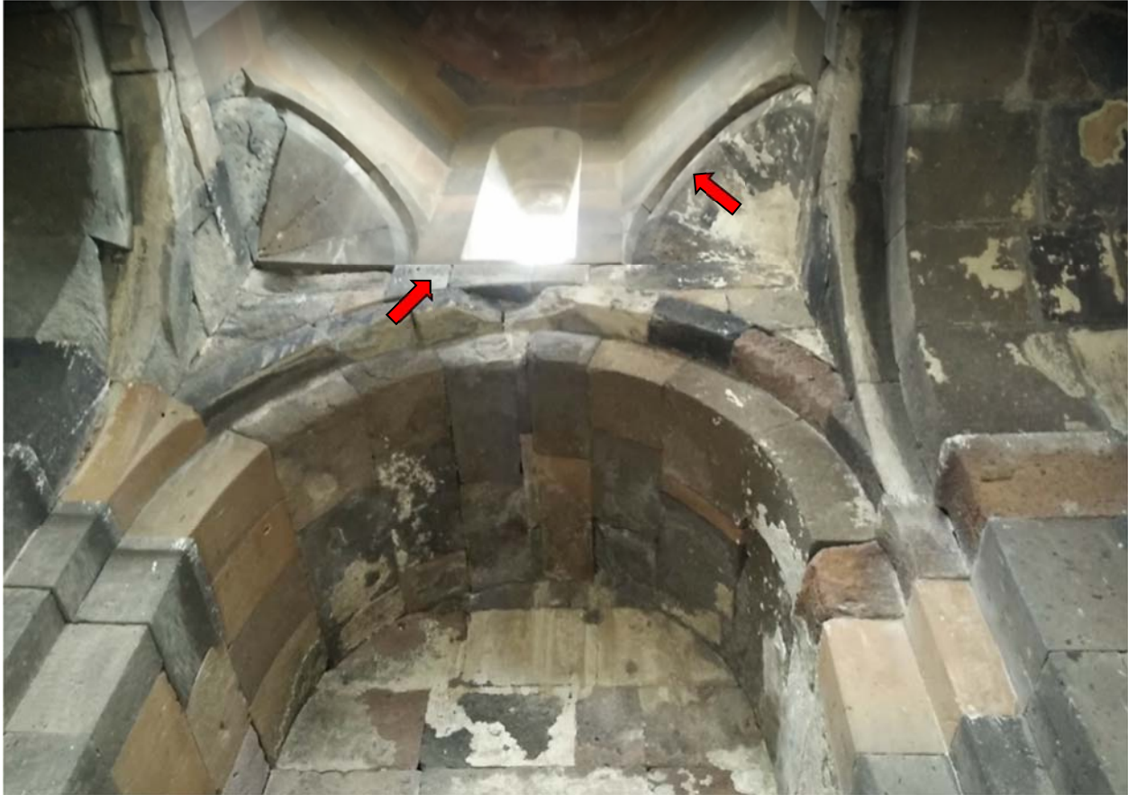
Saint Stepanos Church of Kosh, interior dome view. The line between the restoration project of 1974-76 and the recently built dome is highlighted.
