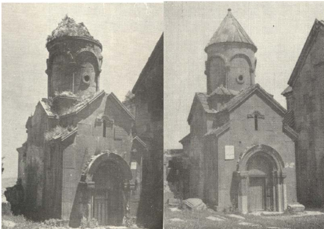
Surb Harutyun Church of Kecharis before and after the restoration project of 1957-58. The missing stones of upper layers, the cornices, the roofs and the dome cover were restored.
