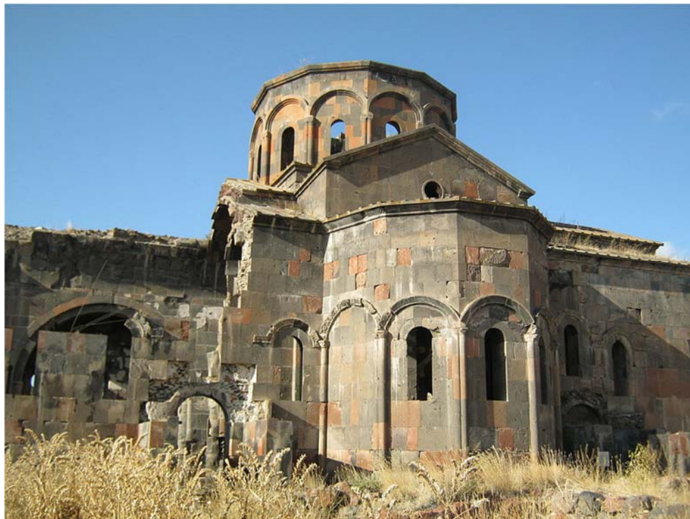
As the monument was heavily damaged, any restoration project would have included using a large amount of new masonry. In this case, the upper sections of walls, the pediments, the cornices and roofs are all restored from new masonry. Photo by Travis K. Witt.
