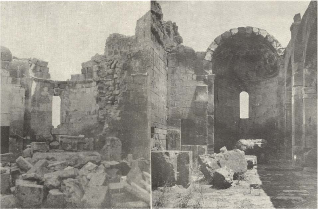
Tsiranavor Church, before and after the restoration project of 1963. The area was cleaned and the apse and the southern abutments were reconstructed using recovered stone blocks.
