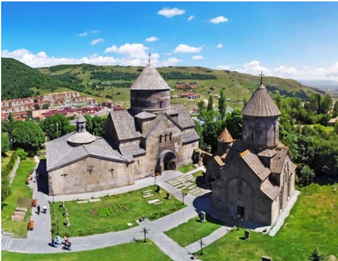
Kecharis Complex in 2015. The domes are reconstructed by unrecognizable stone masonry. Photo by Vahagn Mosinyan, October 2015.
