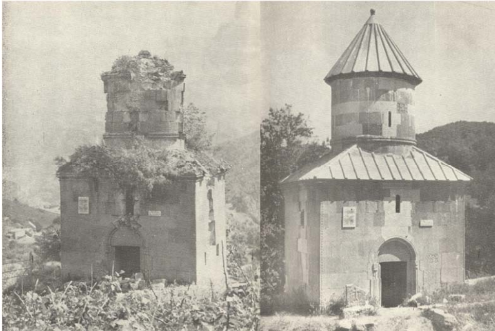
Goshavank, Surb Grigor Church, before and after the restoration project of 1957-59. The missing stones are replaced by new ones but in different color, the roofs are restored and the dome covering which was completely lost was restored by new stone slabs.
