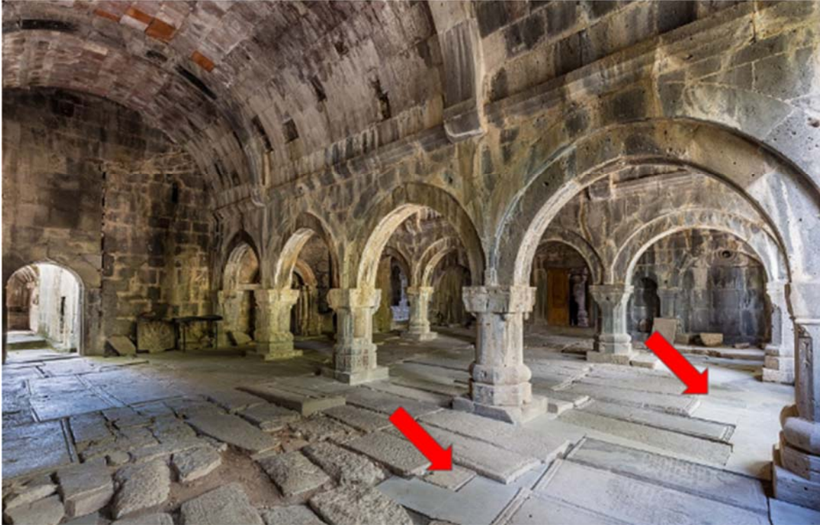
General view of the narthex after the addition of the new pavement. Photo taken on 30 September 2016 by Diego Delso.
