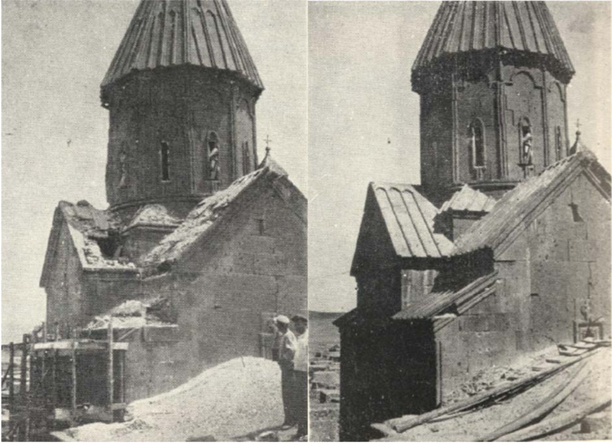
Surb Mariane Church before and after the restoration project of 1950. The missing stones, cornices, and roofs were restored.
