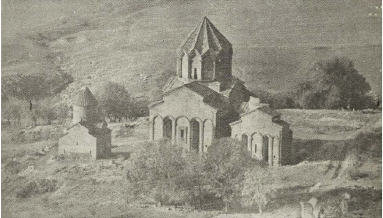
Marmashen Monastery before and after the restoration project of 1954-55. The church located on the North of the main church was the most damaged one. The eastern elevation was completely lost together with part of the northern elevation, vaults and the dome. These lost segments were not reconstructed, the masonry was consolidated. The lost pediments and roofs of the southern church was restored.
