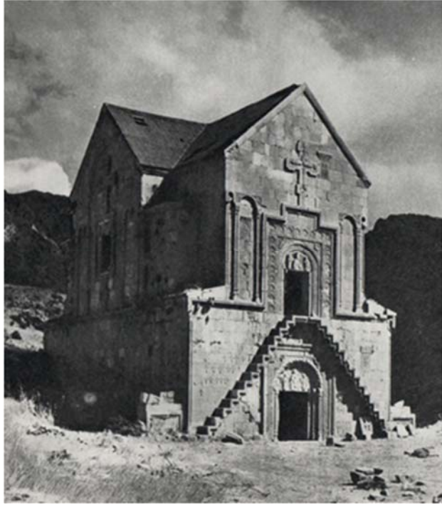
Surb Astvatsatsin Church in Noravank Monastery after its walls preservation.
