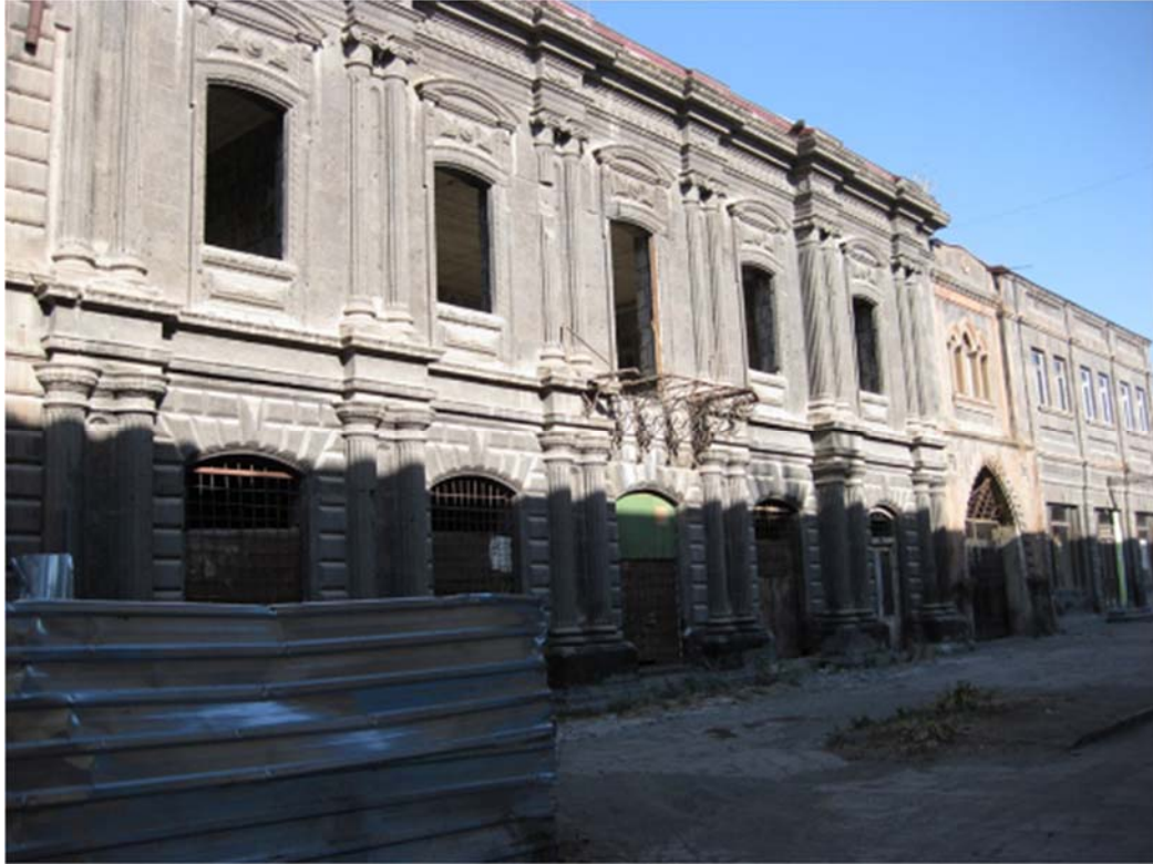
An example of nineteenth century stone architecture in Gyumri during the restoration activities. Photo by Marco Brambilla.
