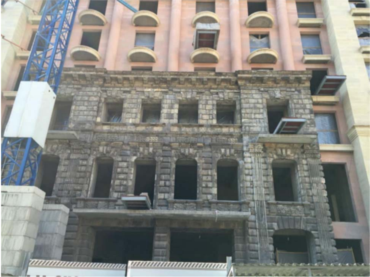
An example of constructing high-rise buildings by keeping the original nineteenth century facade.
