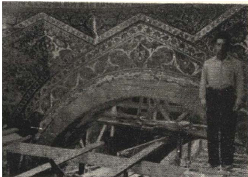
Figure 9: Strengthening of the main arches under the dome by steel reinforced concrete. . Image from Hovhannisian, Konstantin. The Restoration of Architectural Monuments in Soviet Armenia , Yerevan, 1978, p. 95.
