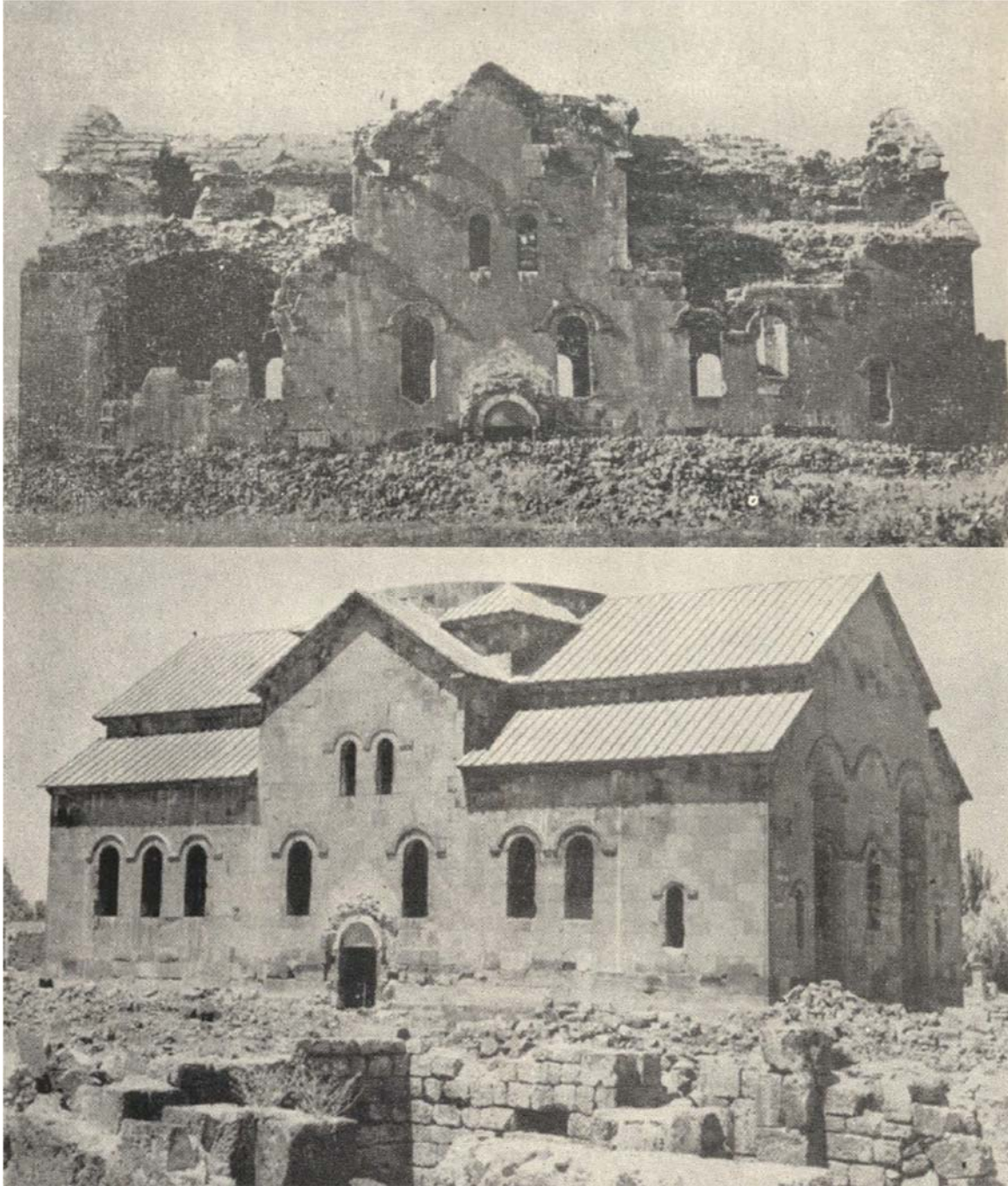
Aruch Surb Grigor Church before and after the reconstruction project of 1958. Both eastern and western vaults are covered by a 20 cm diaphragm of steel reinforced concrete to consolidate the stone blocks. The missing stones of the walls are restored and the roofs are covered by stone slabs. The dome is not reconstructed.
