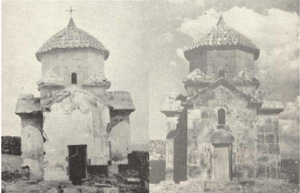
Karmravor Church during and after the restoration project of 1956.
