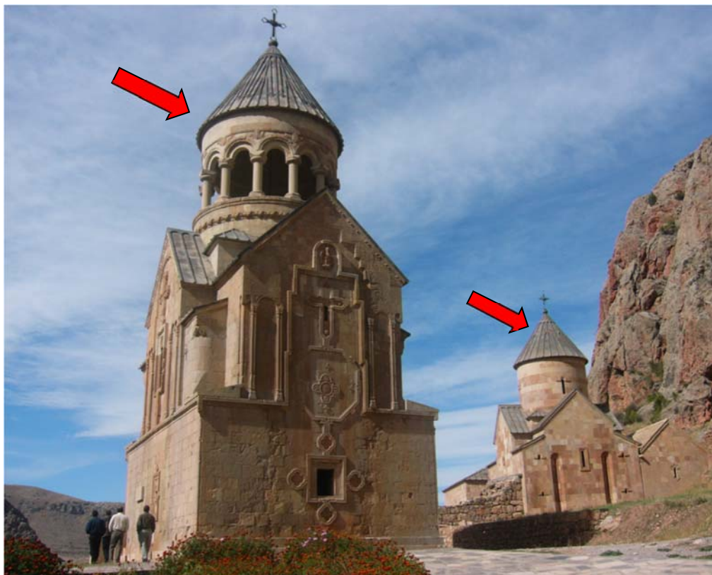
The two recently constructed rotunda and dome in Noravank Monastery. The complex was suggested for entering the list of the World Heritage Sites of UNESCO but was denied due to heavily and not authentic reconstructions.
