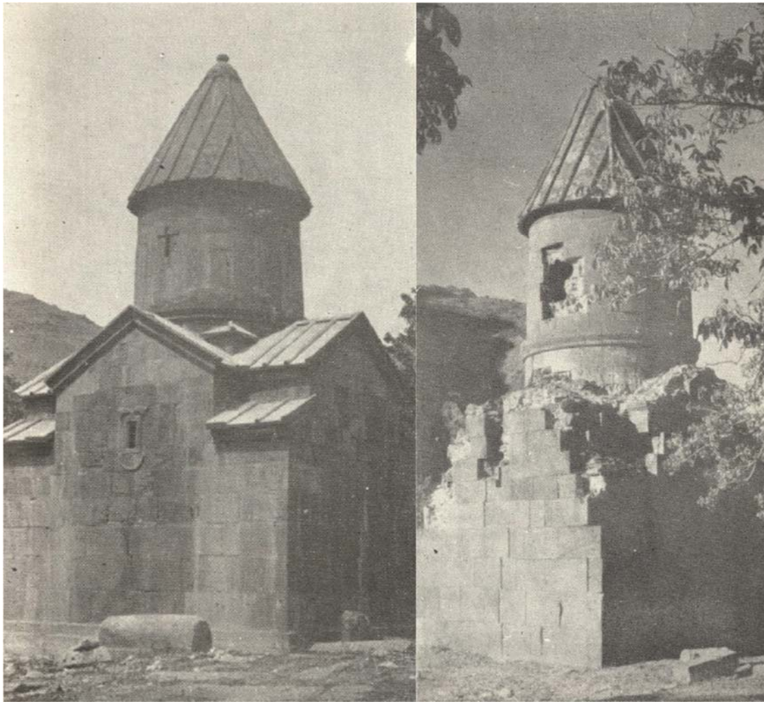
Surb Nshan Church in Yeghegis, before and after the restoration project of 1974. The upper section of the walls, the pediments, cornices, roofs, drum and dome were restored.
