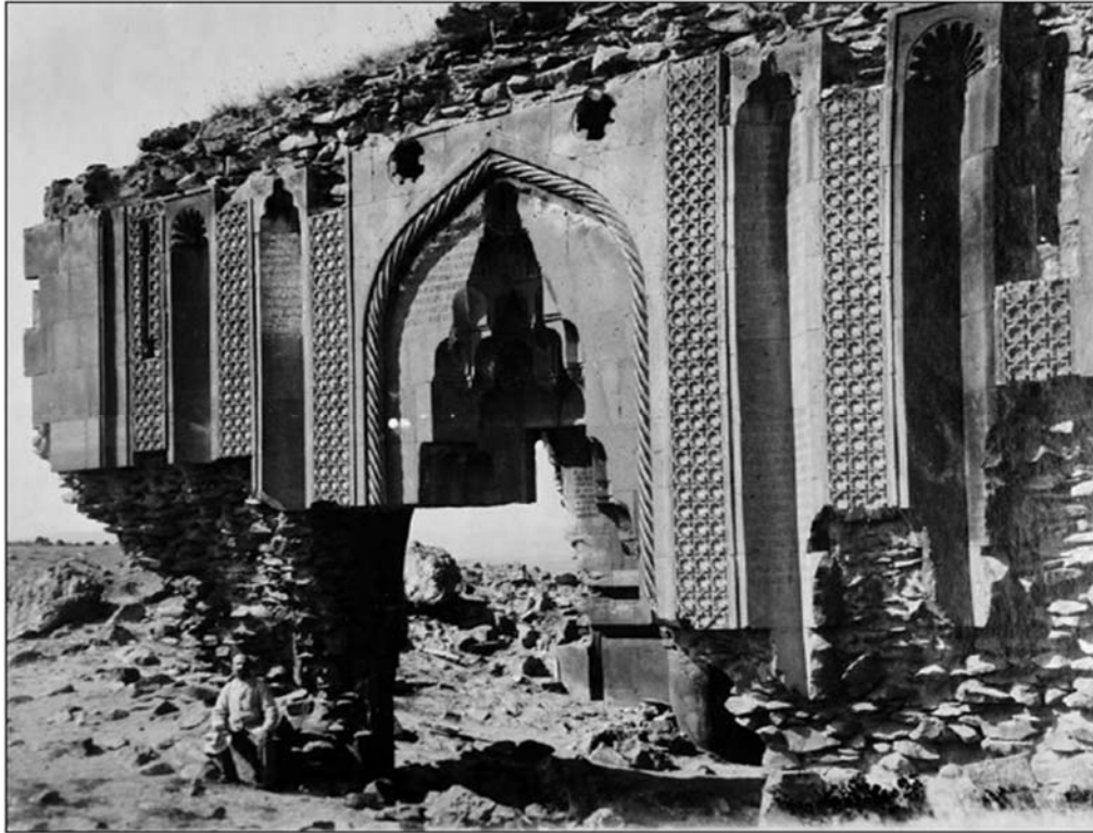
Figure 7: The facade of Holy Apostles Church (Surb Arakelots) at Ani before its partial preservation intervention. Photo from Karapetyan, Samvel. Ani-1050 , Yerevan: RAA, 2011, p. 116.
