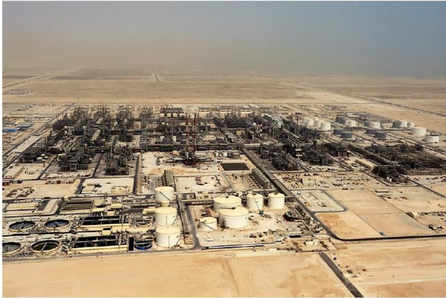
Figure 32. Aerial view of Pearl GTL plant. (41)
