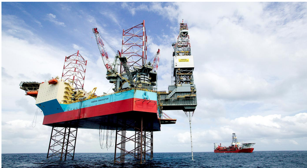
Figure 4.3: Offshore fixed platform
