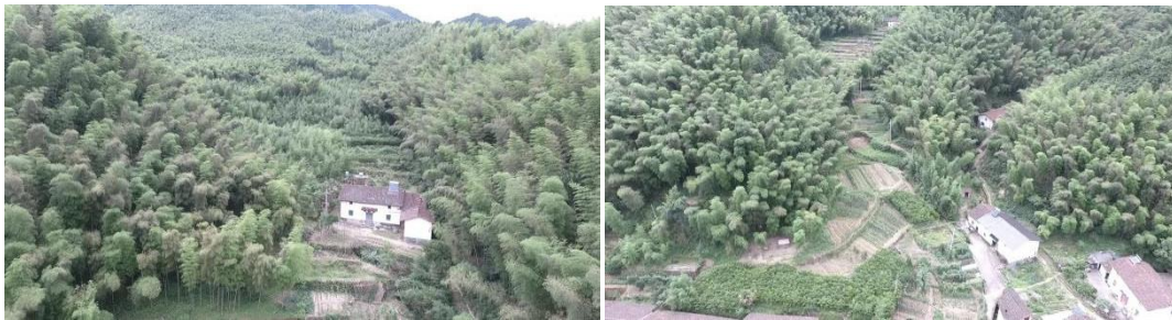
Figure 3.5 Bird's-eye view of the original building
