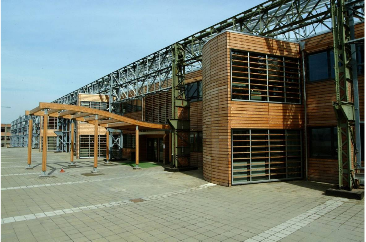
Figure 44 - View of the service center, main building of the Environmental park of Turin
