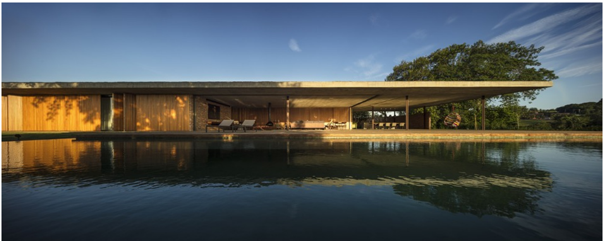
Figure 71 - Casa Plana frontal view
