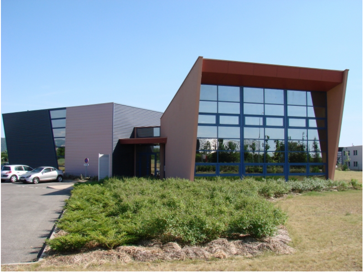
Figure 51 - Perspective view of some buildings of the Parc Industriel Plaine de l'Ain
