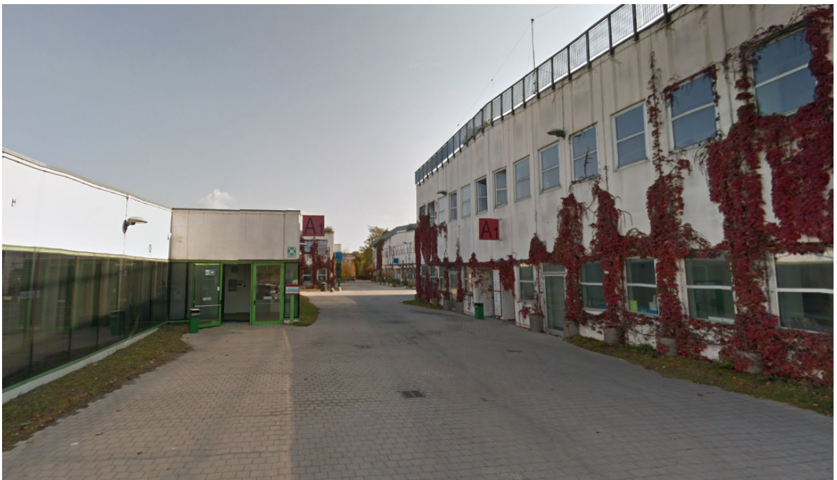
Figure 43 - Perspective view of some buildings that make up the Environmental park in Turin
