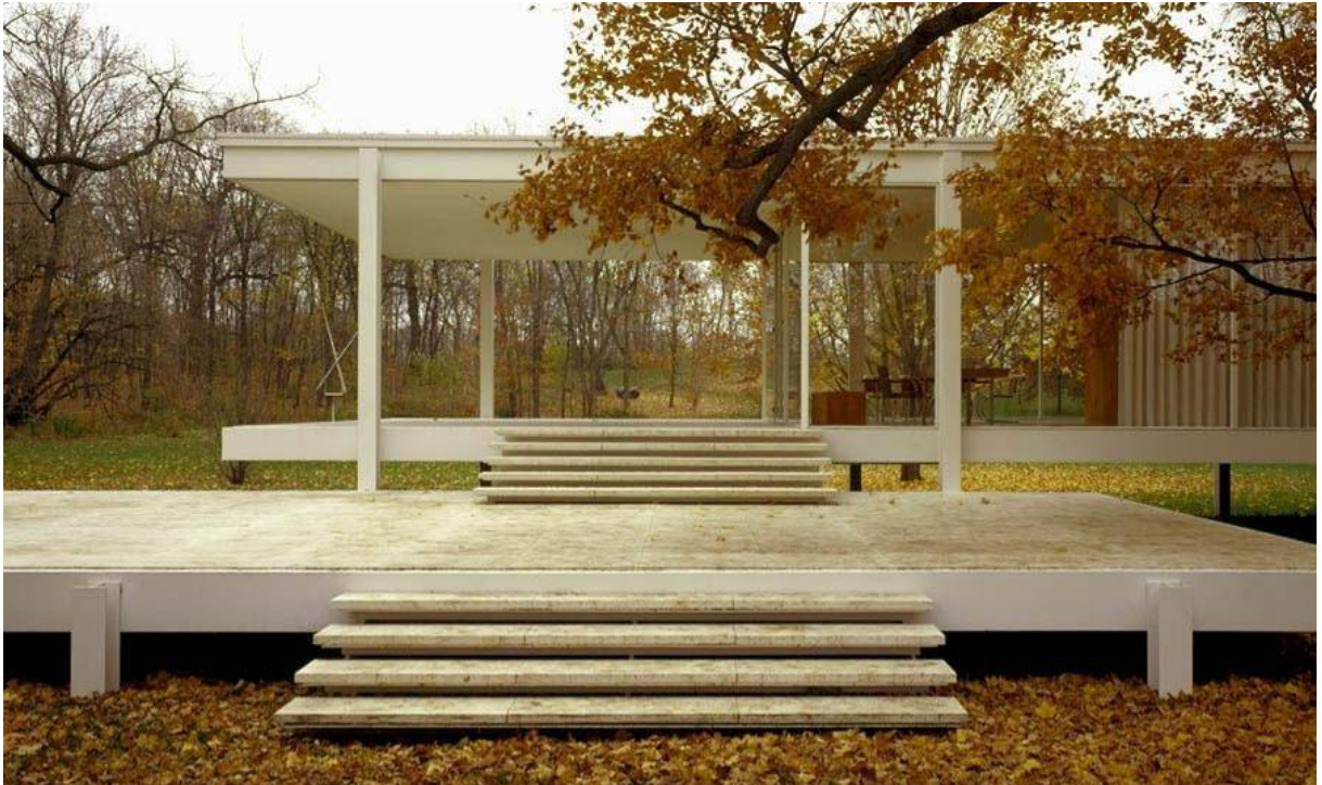
Figure 77 - Farnsworth house entrance
