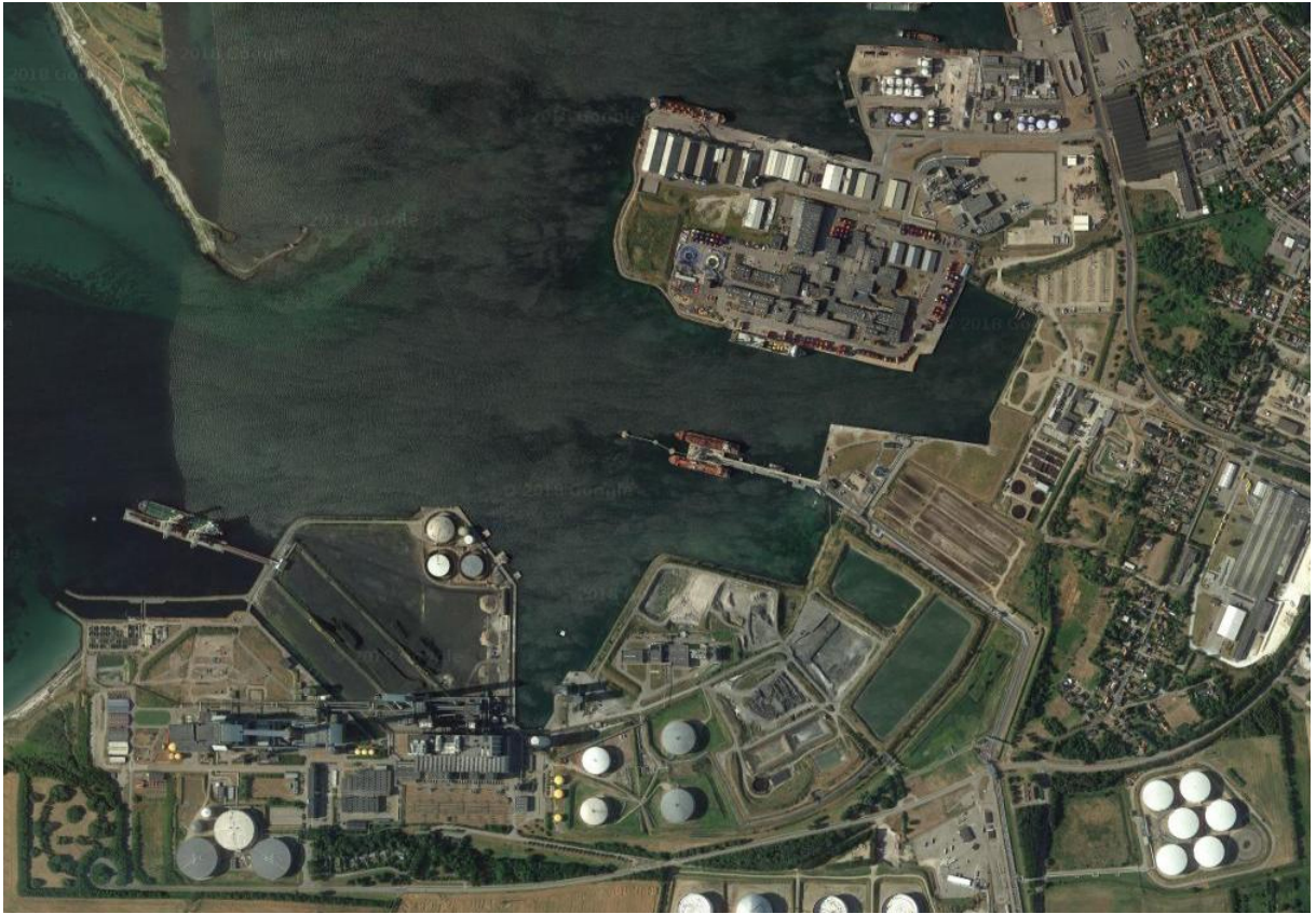
Figure 58 - Aerial view of the Kalundborg industrial park's buildings
