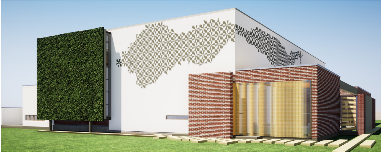
The facade shows the tema designs applied to the white washed walls using a stencil and paint brush to imitate the undulating hills of Maseru.
