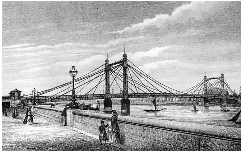
Figure 1.2 : First use of cable-stayed technology. Veranzio concept (top) – Albert Bridge (bottom)
