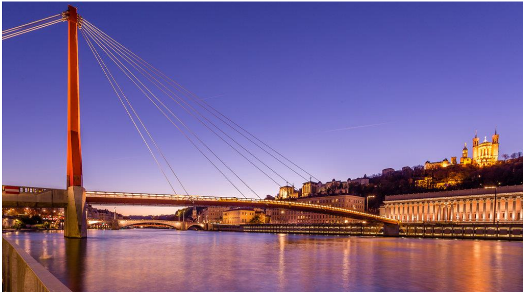
Figure 1.10 : Palais-de-Justice footbridge, France
