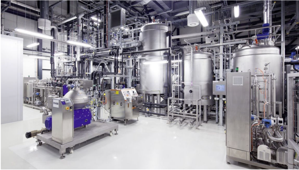
Figure 4: Partial view of the AUDI e-fuel plant.
