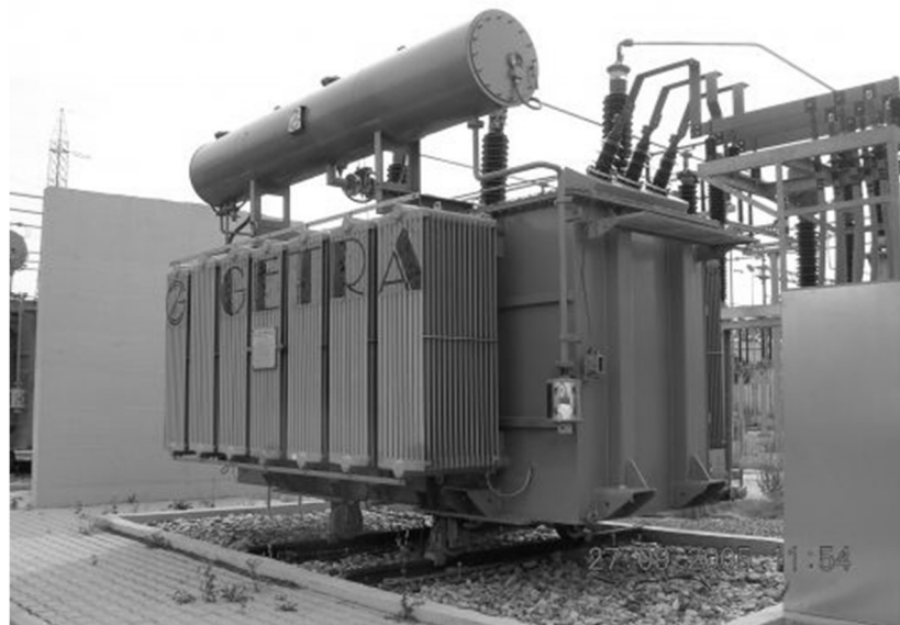
Figure 2.5 Power transformer
