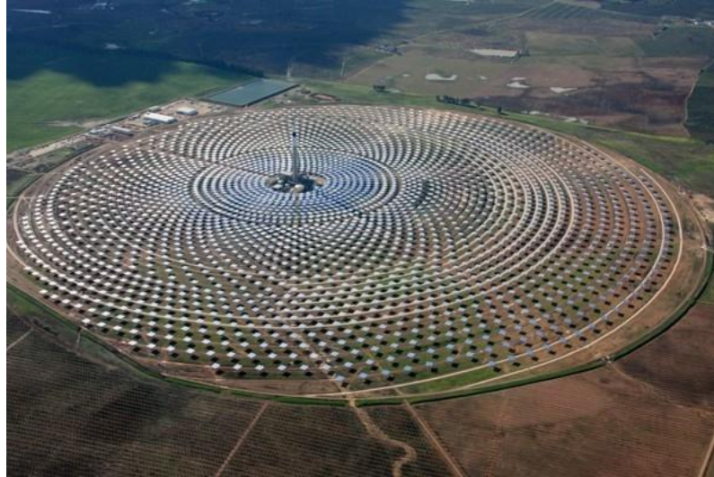
Figure 2.13: Gemasolar heliostat field layout
