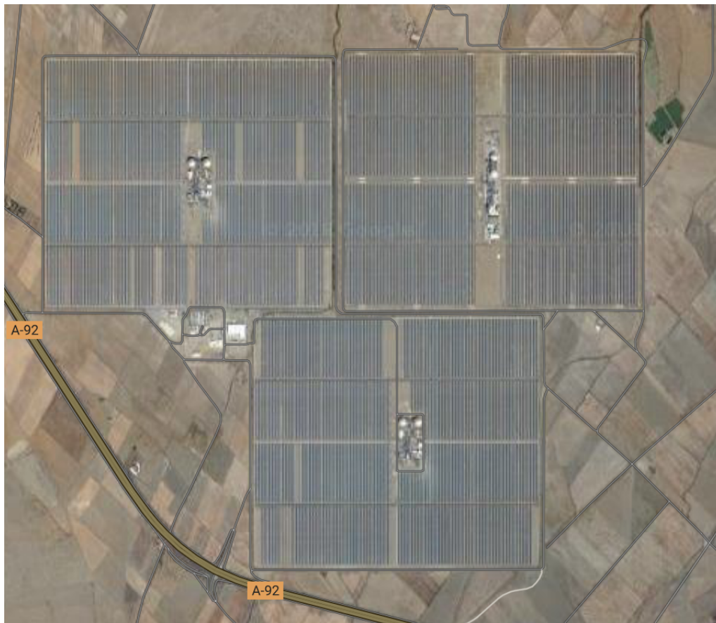
Figure 19: Andasol I, II and III
