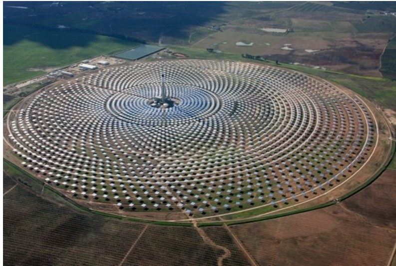
Figure 2.12: Gemasolar heliostat field layout
