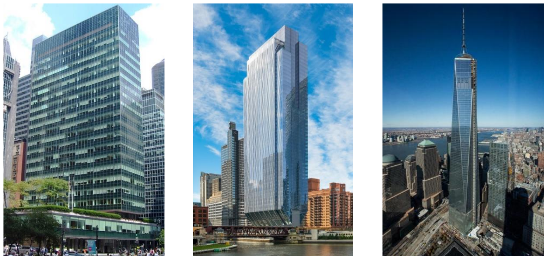
Figure 2.11: Lever House (Rigid Frame); North Riverside (Shear Walls); World Trade Centre (Outriggers)
