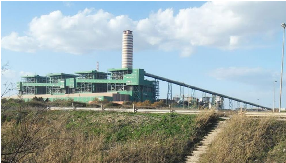
Figure 4.1 Federico II power plant
