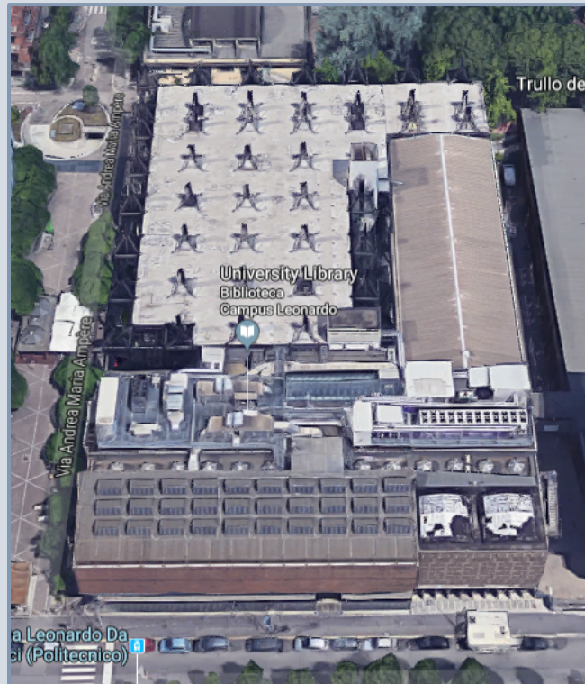
FIGURE 17 - BUILDING 11 ARCHITECTURAL BUILDING (COURTESY GOOGLE MAPS)
