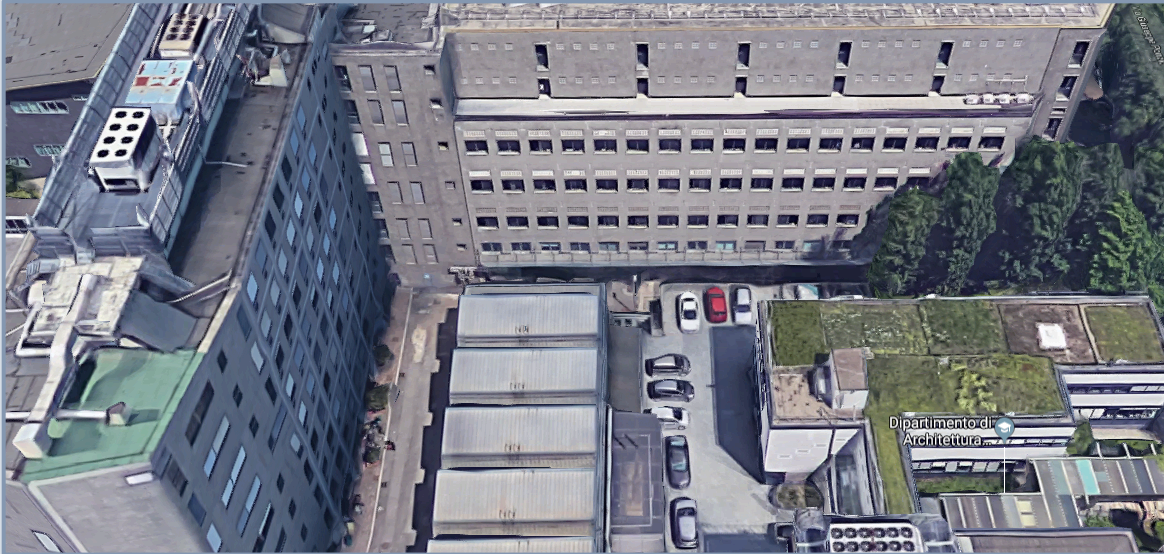
FIGURE 18 - BUILDING 14 NAVE (COURTESY GOOGLE EARTH)
