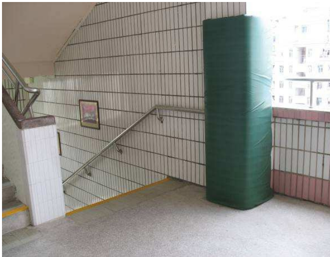
Protection pad of column
