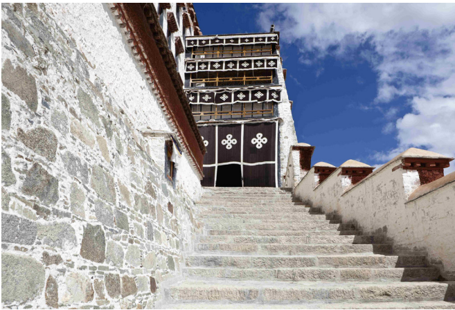
White architectural element in Lhasa
