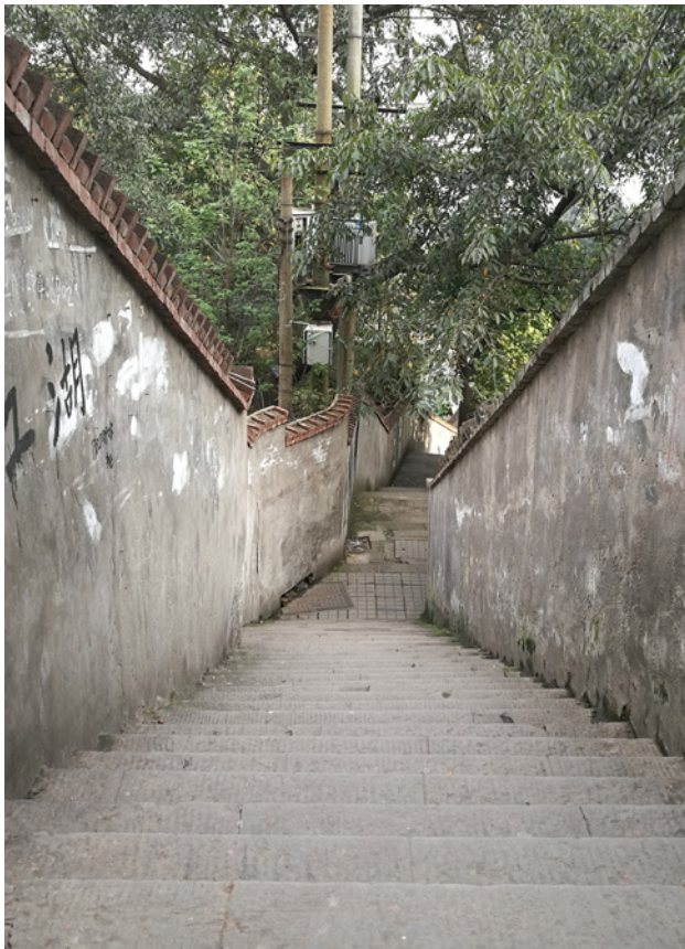
stairs connecting 30m height difference
