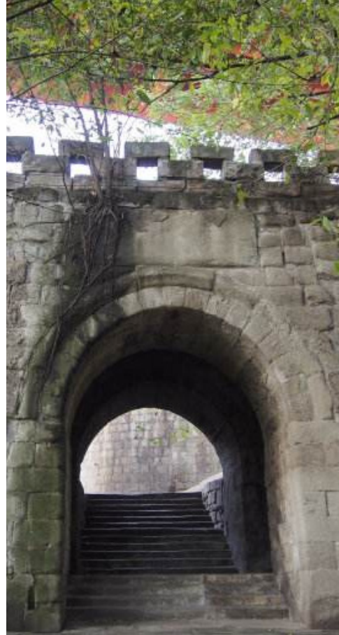
Dongshuimen City Gate under Dongshuimen Bridge
