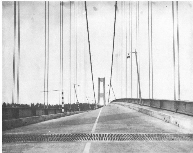
Figure 2.8: Torsional oscillation of TNB seen from a tower. Source: [2].
