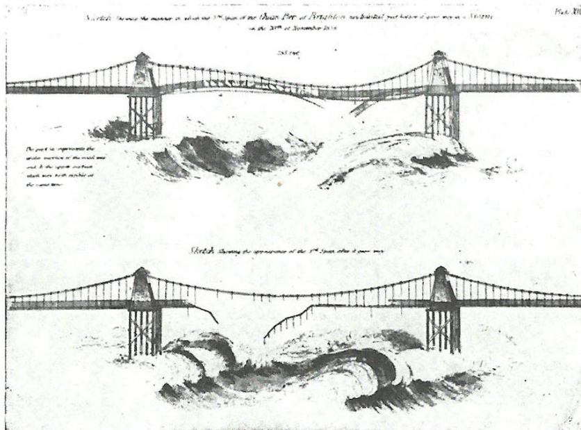
Figure 2.5: The failure of the Brighton Chain Pier (1836) reproduced by W. Reid.
