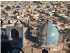
Fig. 4-1 Aerial photo of Shah Mosque's dome. © Photo by Barati 2007
