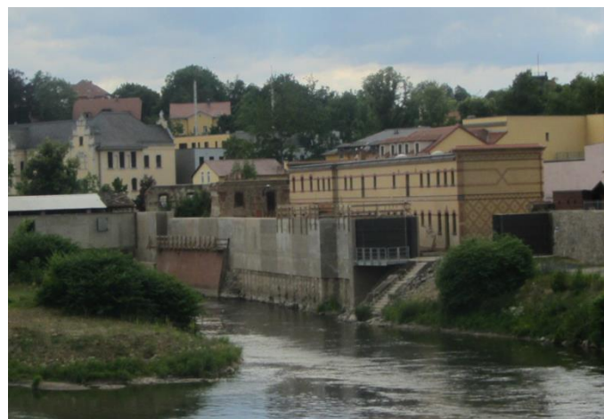
Figure 40 Floodwall, Project 2, under construction in June 2017 (source: author).
