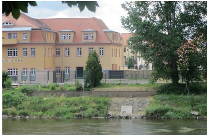
Figure 39 New floodwall, part of Project 2, with passageways for accessing the river and allowing a view (source: author).
