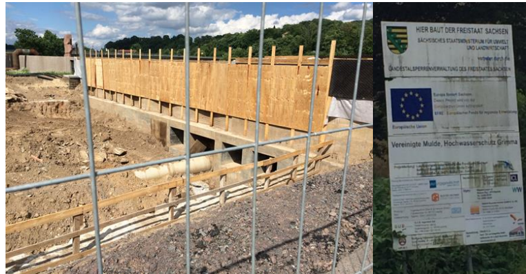
Figure 42 Floodwall, project 4, under construction in June 2017 (source: author).
