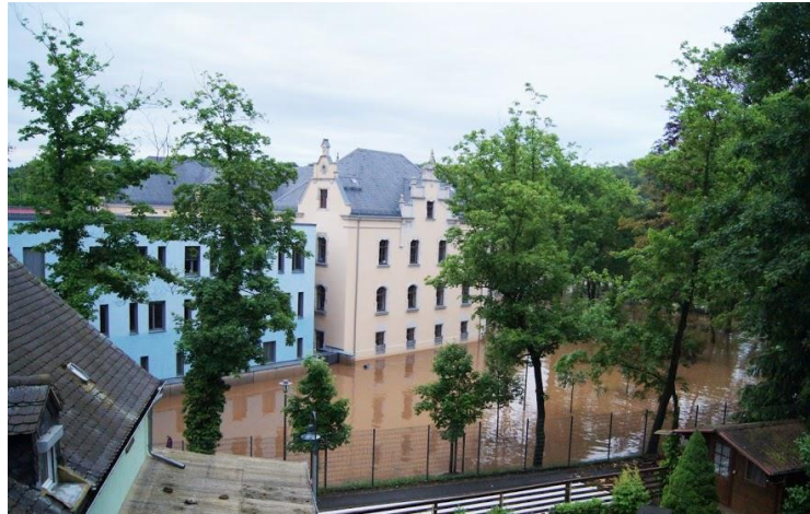
Figure 45 New police station flooded during the 2013 flood (source: Colditzer-tageblatt , 2013)
