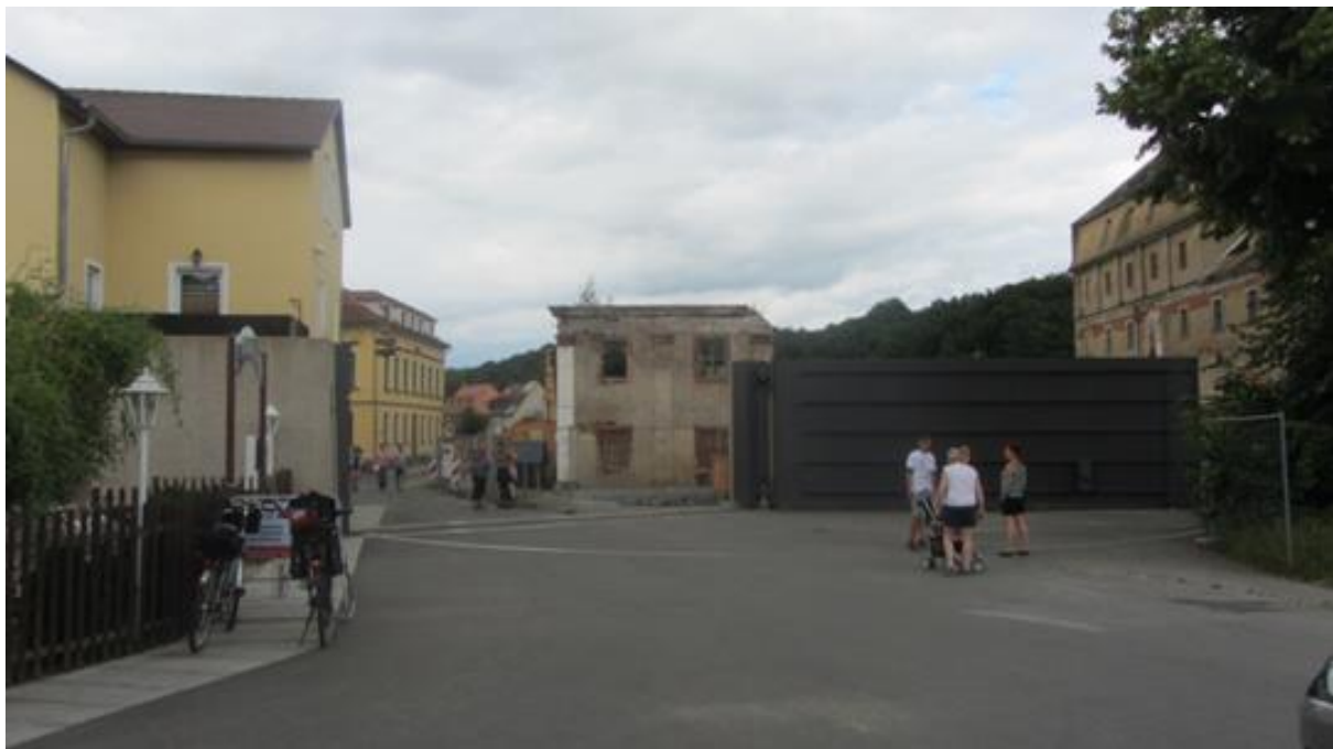
Figure 38 Floodgate, part of the floodwall Project 1 (source: author).
