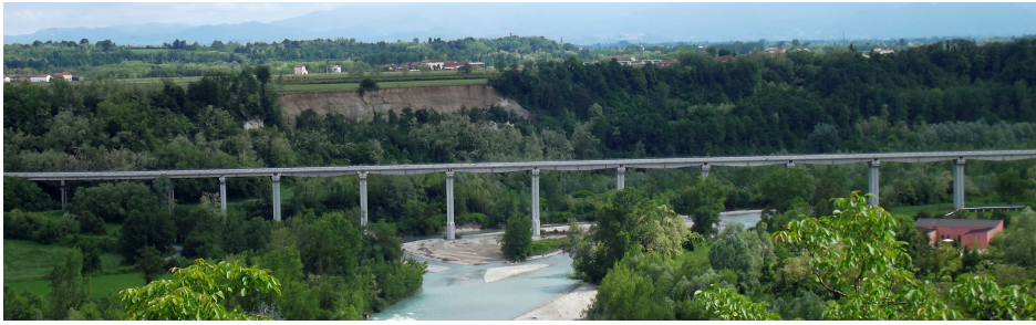
(a) View of the bridge.
