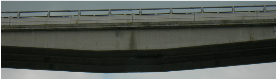
(a) View of the bridge.
