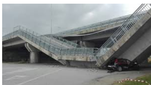
(b) Fossano Bridge.
