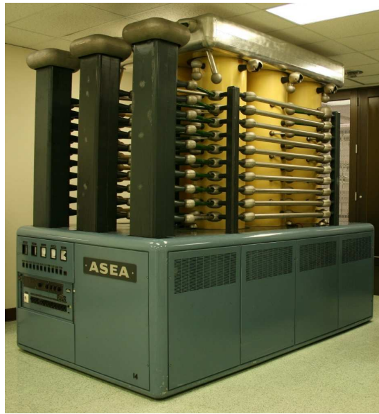
Figure C.26: ASEA-design Mercury-arc rectifier installed in Pacific Intertie project (United States of America, 1970. Source: ABB).
