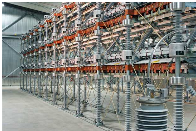
Figure C.28: IGBT-based modules for HVDC converter.
