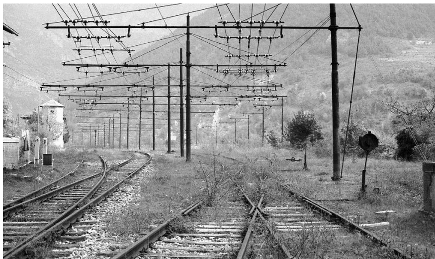
Figure C.18: Three-phase catenary at Vievola (France, 1970, the very last period of three-phase railway. Source: stagniweb.it ).
