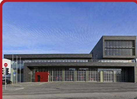
Fire Station in Vilnius | 2012
