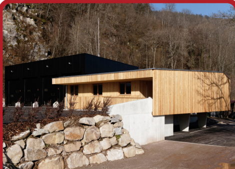
Fire Station of Metzeral | 2017
