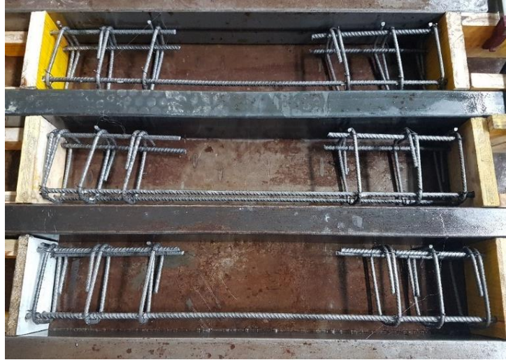
Figure 3–27. Reinforced beams with rebars and stirrups
