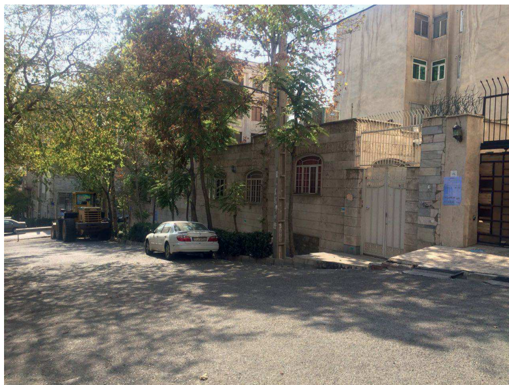
Picture below, south-west view
